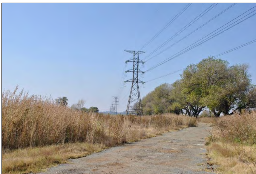
Figure 6-4: Servitude of the power line, road and railway within which the proposed pipelines lay
