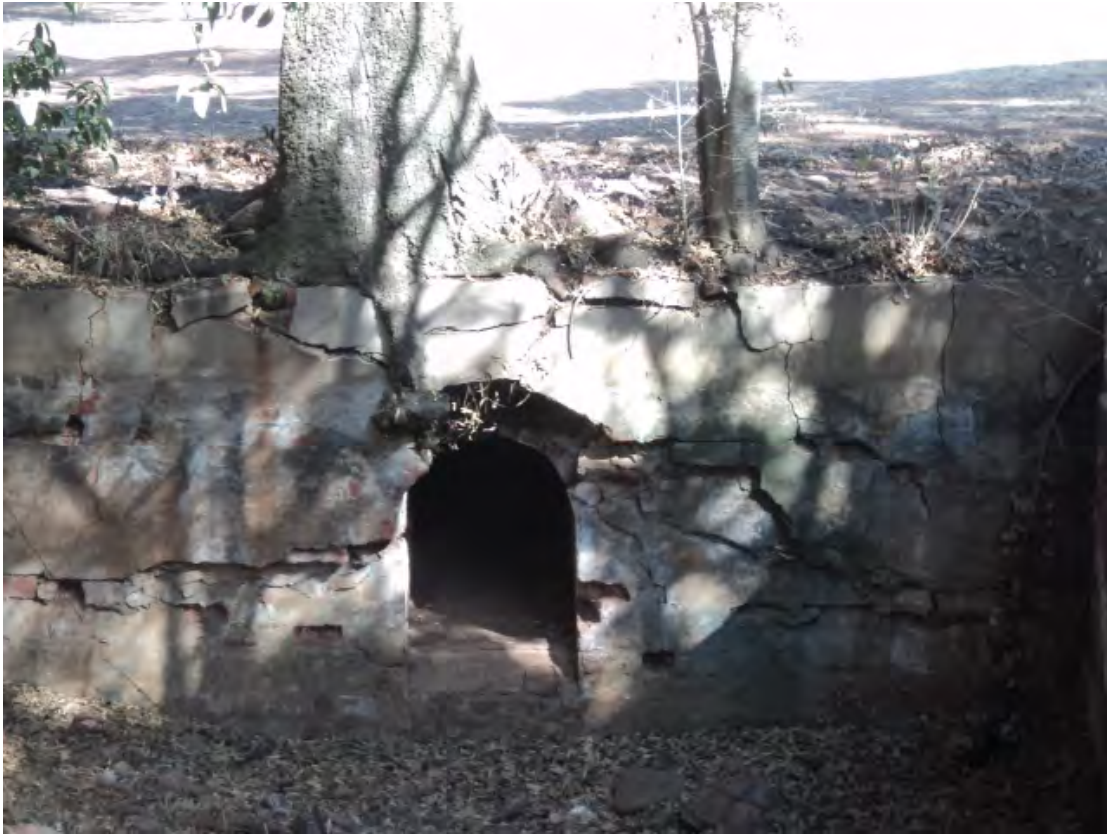
Figure 23. Underground canal and sump.
