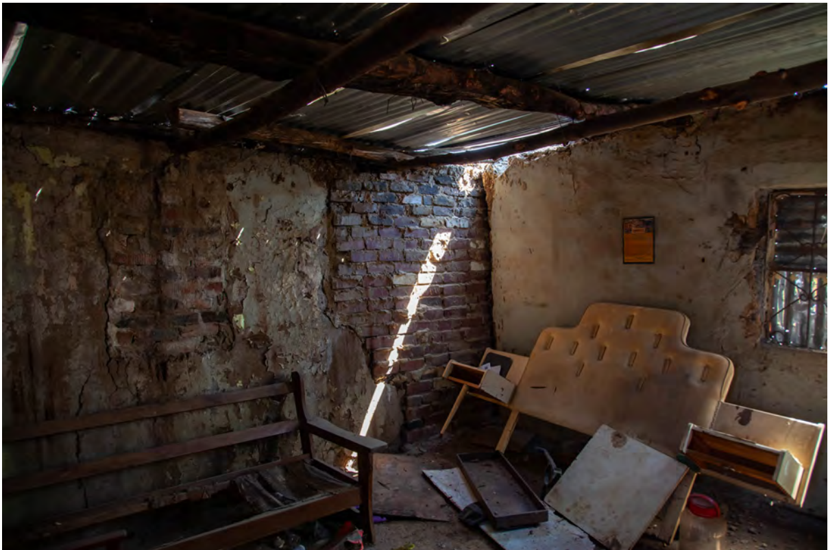
Figure 55. Room in abandoned Manyaka family house at ZK23/2019.
