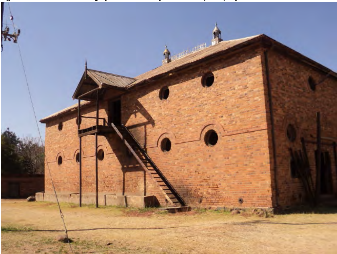
Figure 12. 1915 new-built double storey dairy.
