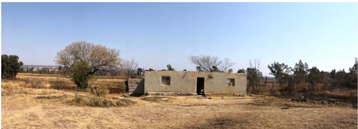
Figure 53. House of the Manyaka family who lived on the farm since the beginning of the 20 th century ZK23 2019.
