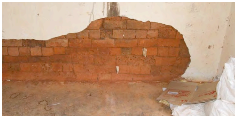
Figure 2 Detail of bricks in old house
