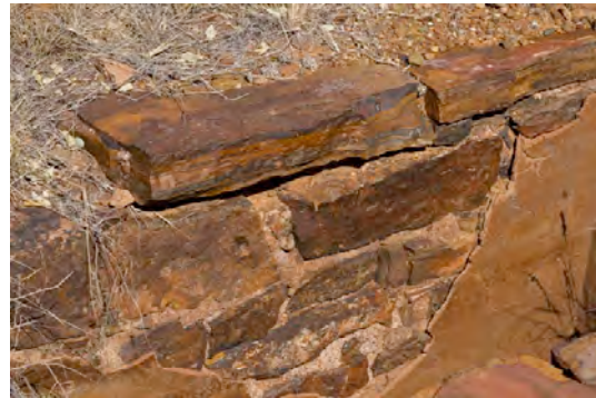
Figure 27 LVW_7a Sheep dip with detail of stone and plaster.
