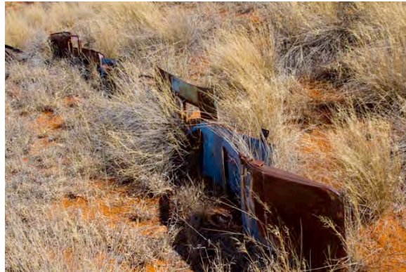
Figure 23 Wall in drainage line constructed of old car doors.
