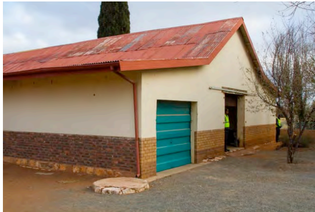
Figure 1 Older house at Heuningkrans
