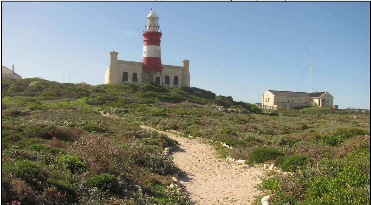
Plate 4: The boardwalk will follow the existing footpath up the hill, terminating at the base of the lighthouse.
