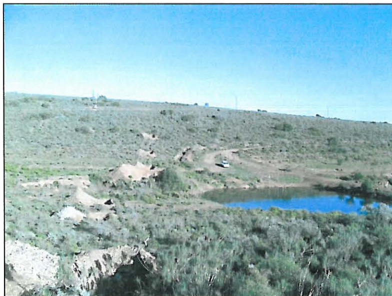
Plate 3: Existing dam. Earth heaps mark geotechnical trials for proposed dam wall
