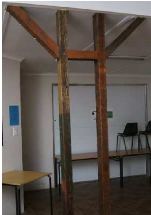
Figure 5. Detail of the joinery where part of the cladding has been removed
