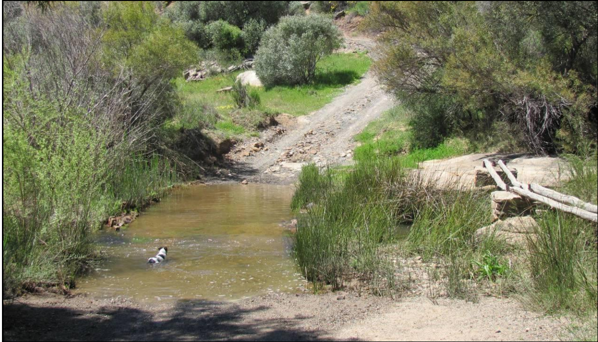
Plate 11: This river will be crossed with a concrete drift while the wooden poles on the right will be replaced with a wooden boardwalk for hikers.
