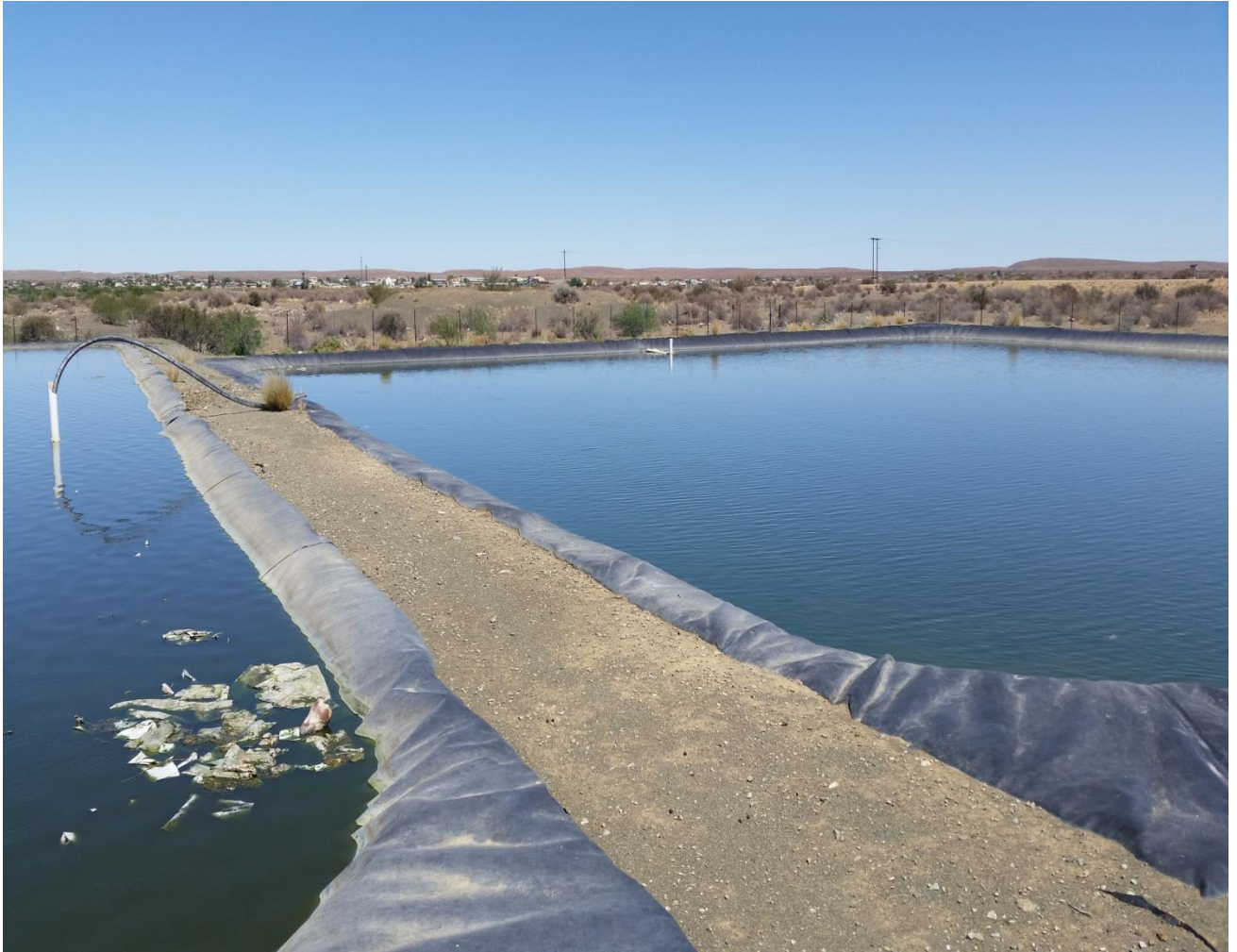
FIGURE 16: Oxidation Ponds to be upgraded at Rietfontein (Two existing ponds)
