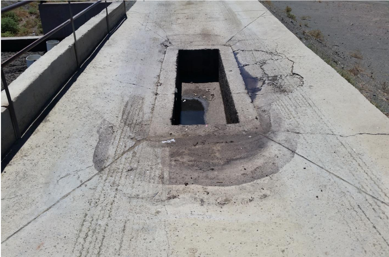
FIGURE 21: Existing Dumping Drain at Rietfontein Oxidation Ponds
