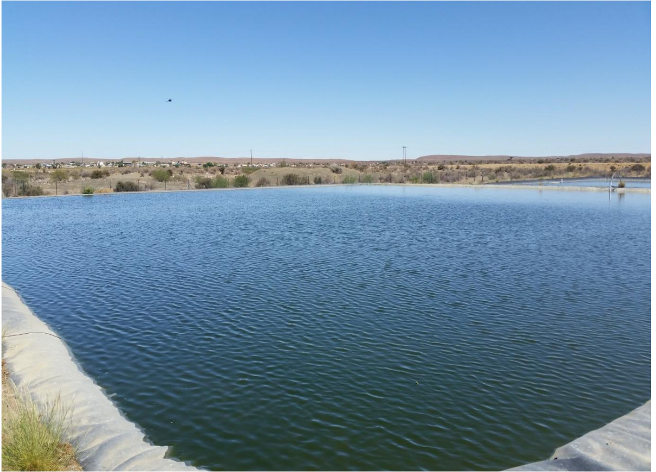
FIGURE 15: Existing Oxidation Pond to be upgraded
