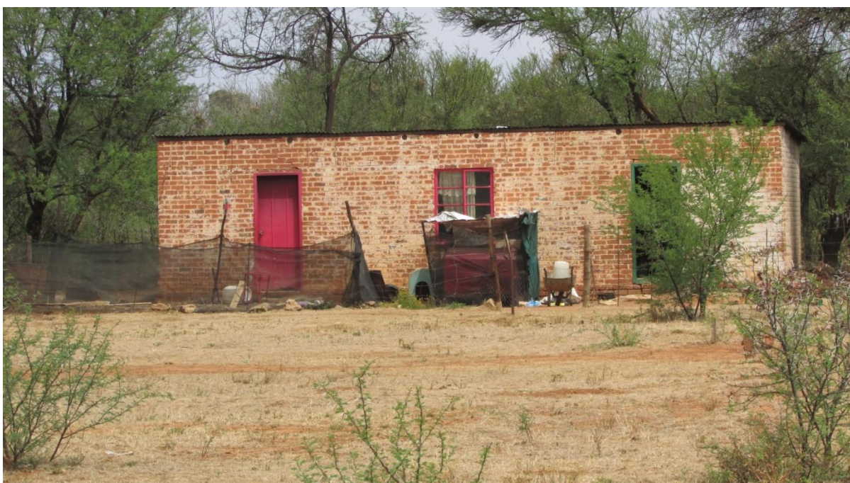
Figure 11: An overview of the last structure noted in the proposed site.
