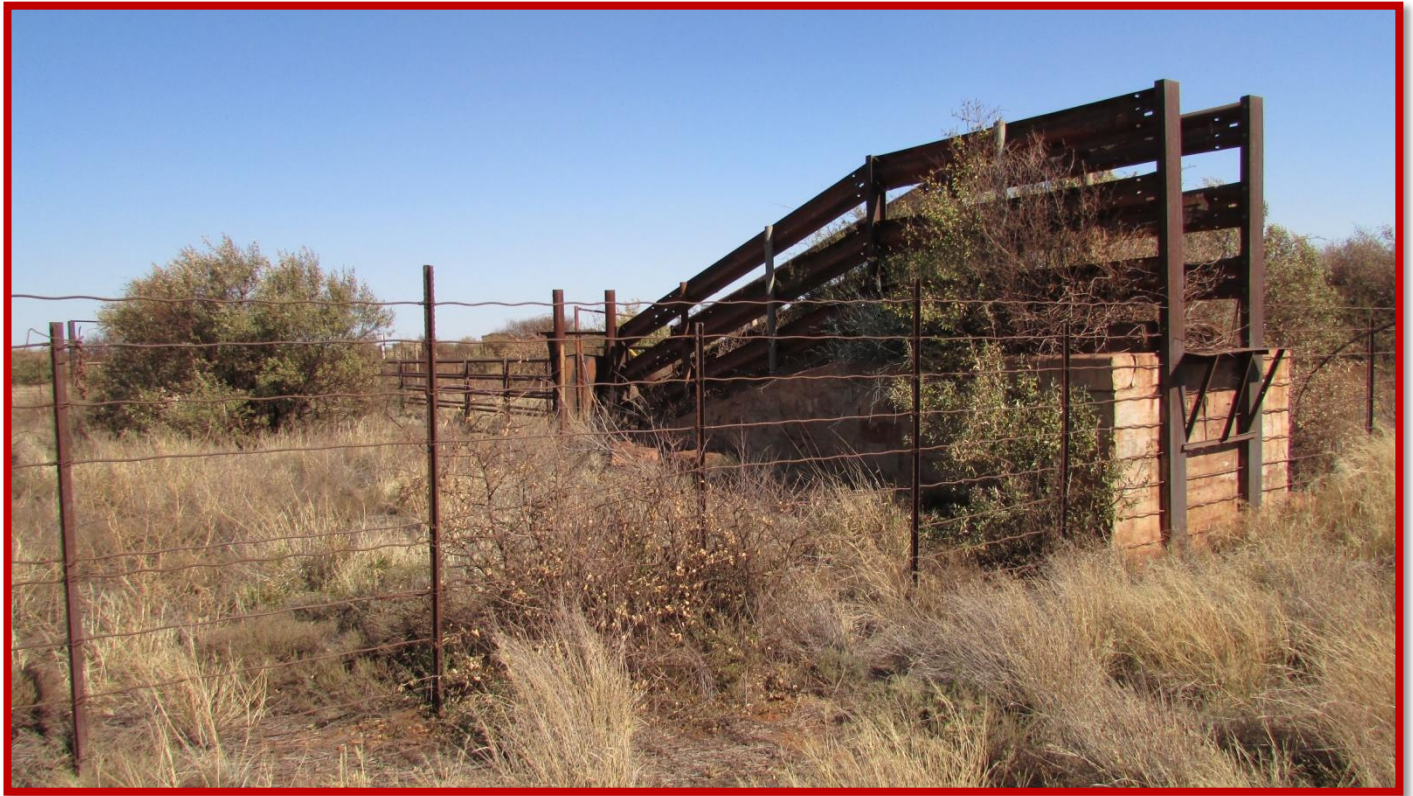
Figure 19: View of the historical cattle pests' maintenance structure.
