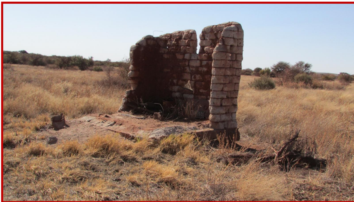
Figure 17: View of the depleted structure constructed of lime bricks.
