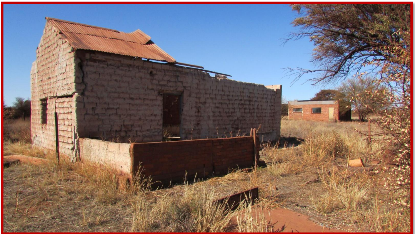
Figure 16: View of structure number two. This structure which is constructed of lime stone is one of the earliest structures in the Northern Cape, and dates to the earliest arrival of the white settlers in the region. Further right of the plate, is another structure which was probably used as a store room for farming equipment.
