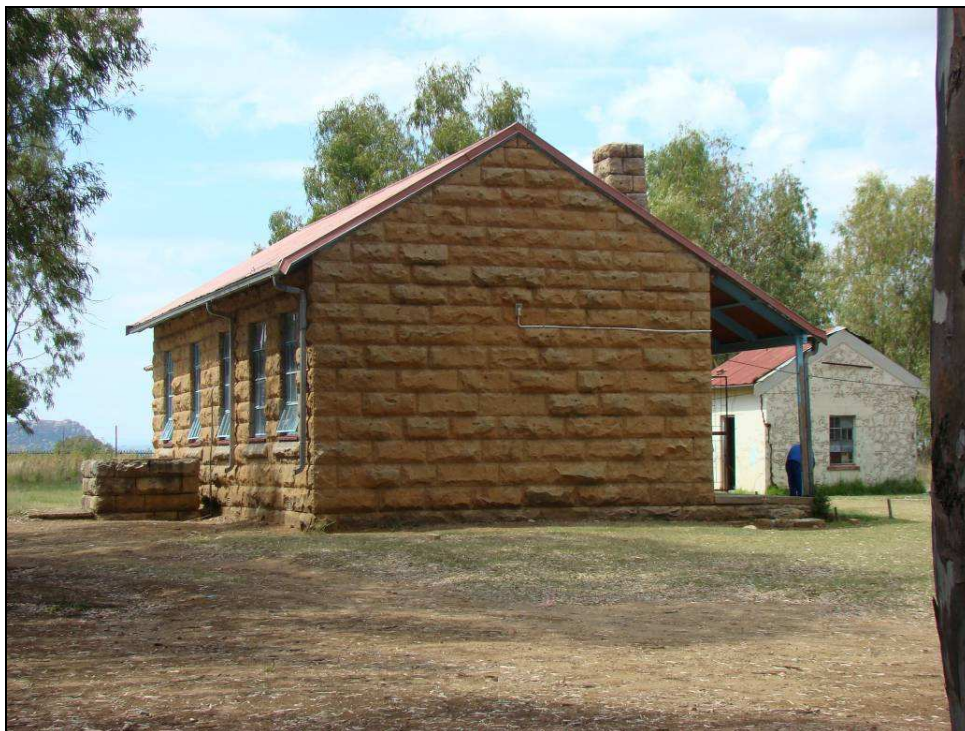
Fig.13 School buildings at Vinies along the S836 road to Maseru.
