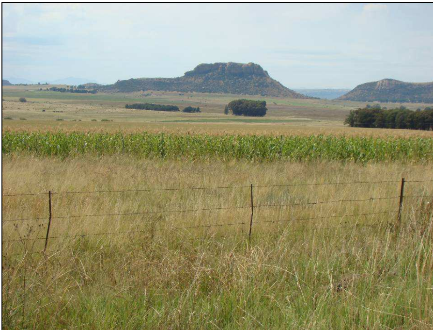
Fig.8 Point D along the S836 gravel road indicating the new route to Maseru.
