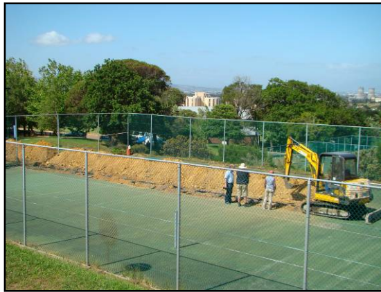
Trench 1: Excavations through the tennis court.
