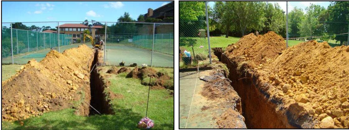
Trench 1, looking north-south (left) and south-north (right).
