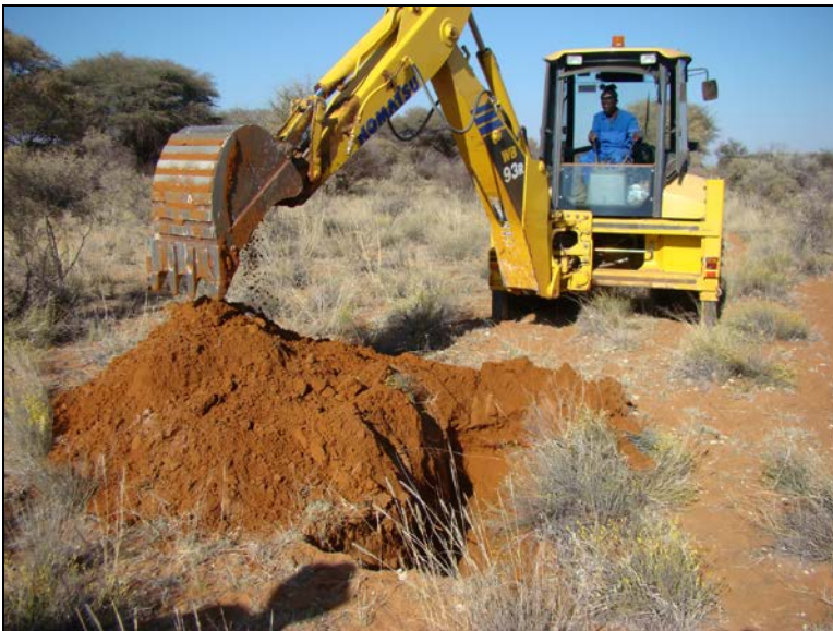
Fig.5 Sterile soil from test pit at Point B.
