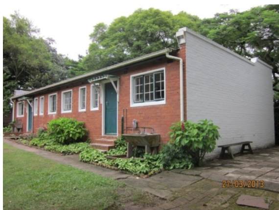
Fig 11: Staff quarters from Labour compound
