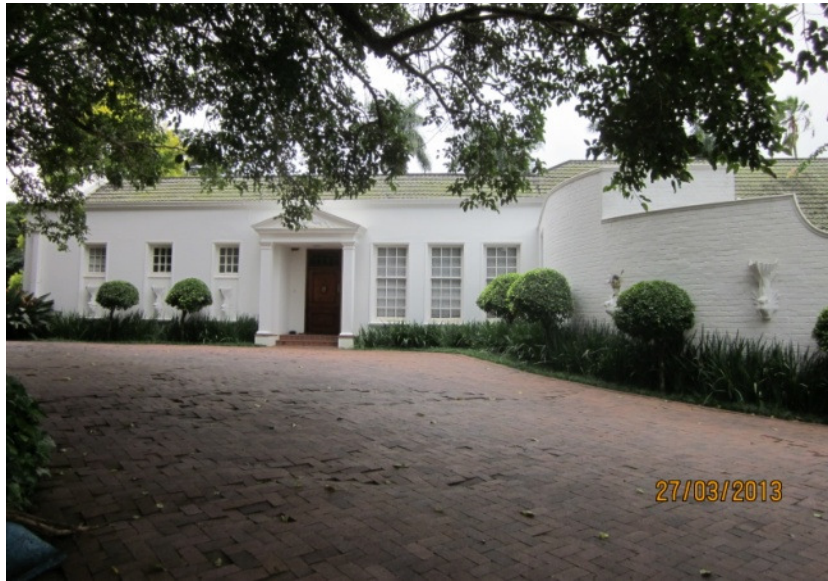
Fig 2: Herrwood House entrance from south west
