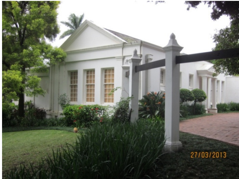
Fig 4: South west façade
