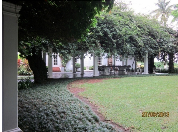
Fig 6: North eastern façade from driveway pergola showing veranda space
