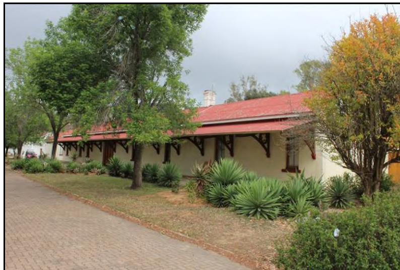
Plate 51: View of the main building of the Site ASU-S36 Colonial Period railway station
