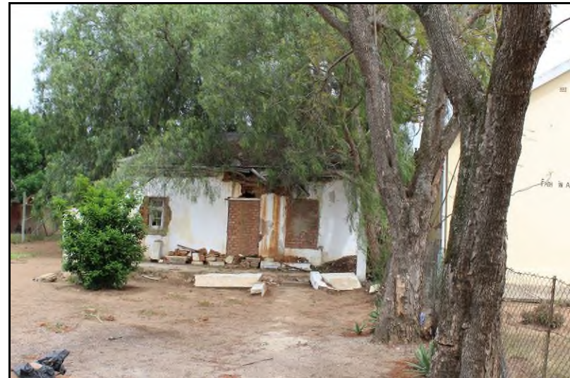
Plate 36: General view of Site ASU-S22
