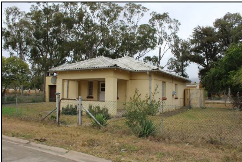
Plate 49: General view of Site ASU-S34
