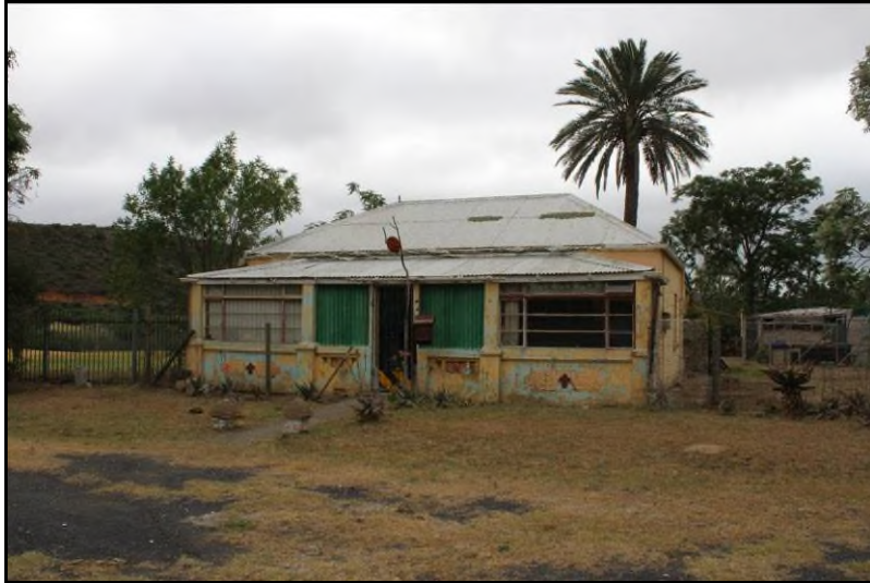
Plate 17: General view of Site ASU-S7
