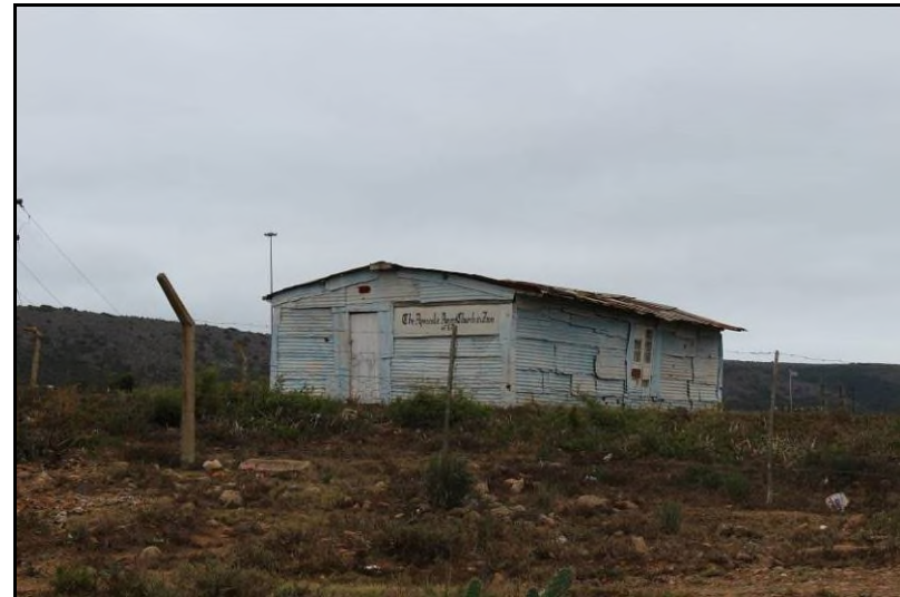
Plate 8: General view of the Site ASU-S3 church building
