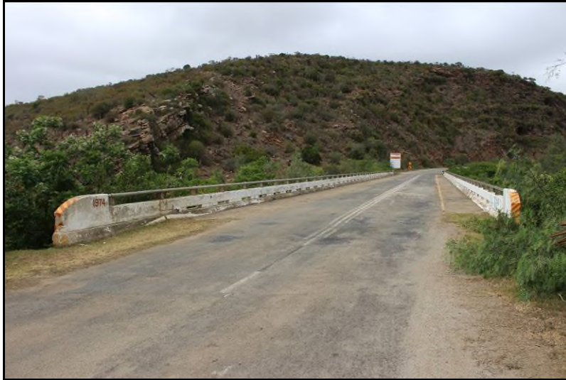
Plate 53: The Site ASU-S38 Contemporary Period bridge
