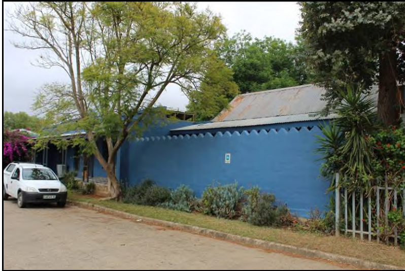
Plate 33: General view of Site ASU-S19
