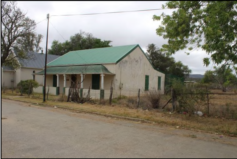
Plate 25: View of the Site ASU-S11 Colonial Period residence
