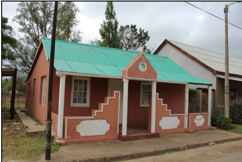
Plate 30: General view of Site ASU-S16
