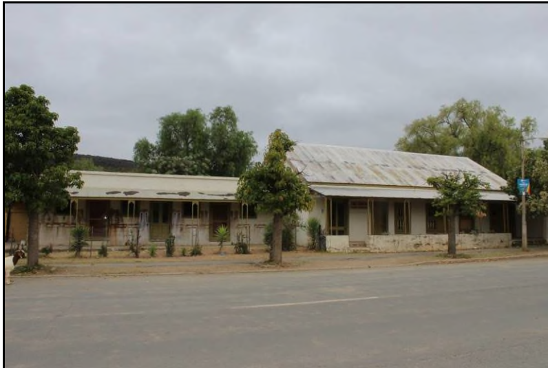
Plate 22: General view of Site ASU-S9
