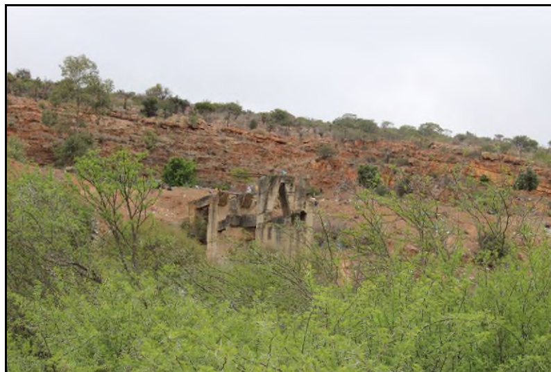
Plate 52: Site ASU-S37 – Colonial Period quarry structure remains
