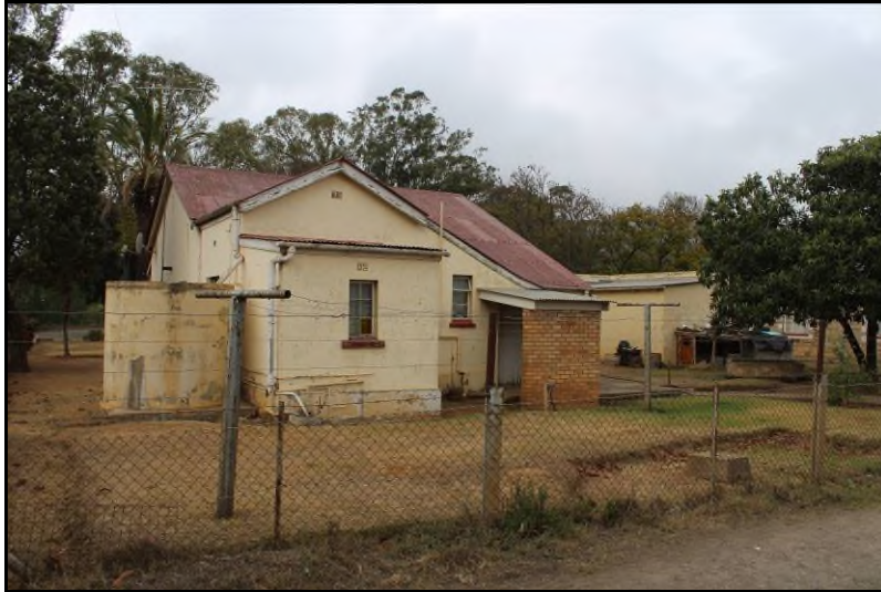
Plate 41: General view of Site ASU-S26
