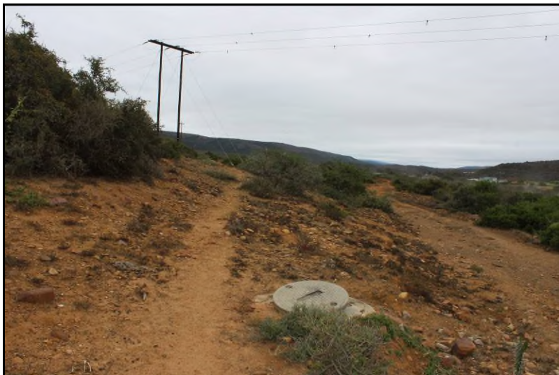
Plate 1: View of the existing sewerage alignment
