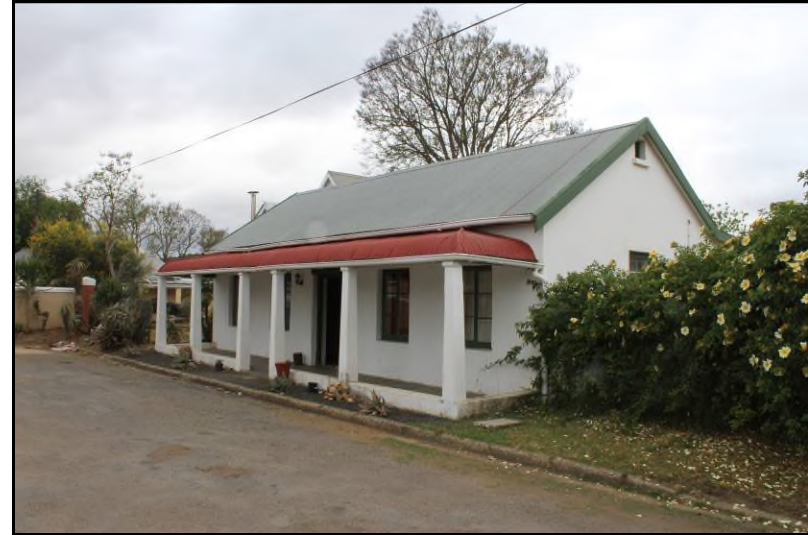
Plate 39: General view of Site ASU-S24
