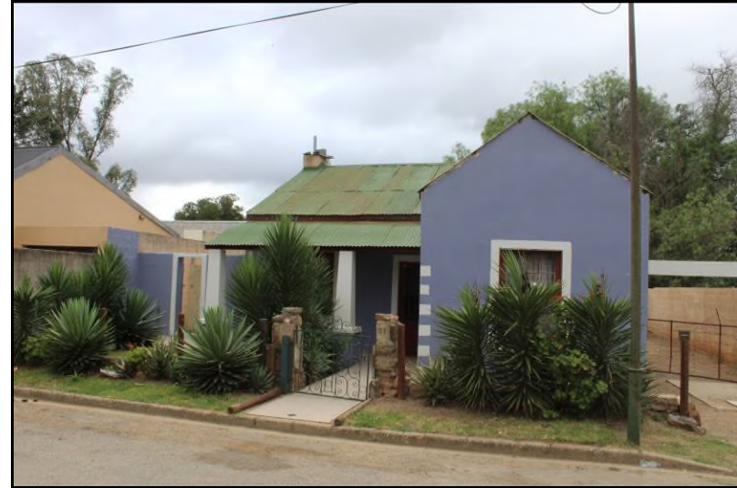
Plate 27: General view of Site ASU-S13
