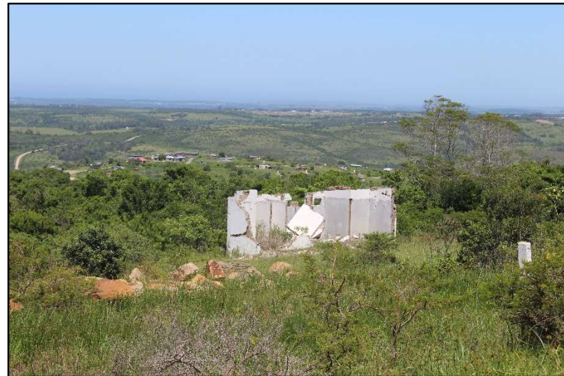
Plate 12: View of Site BWD-01 structure remains adjacent to the reservoir
