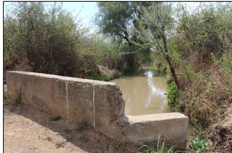
Plate 9: View from the bridge across the flood irrigation system
