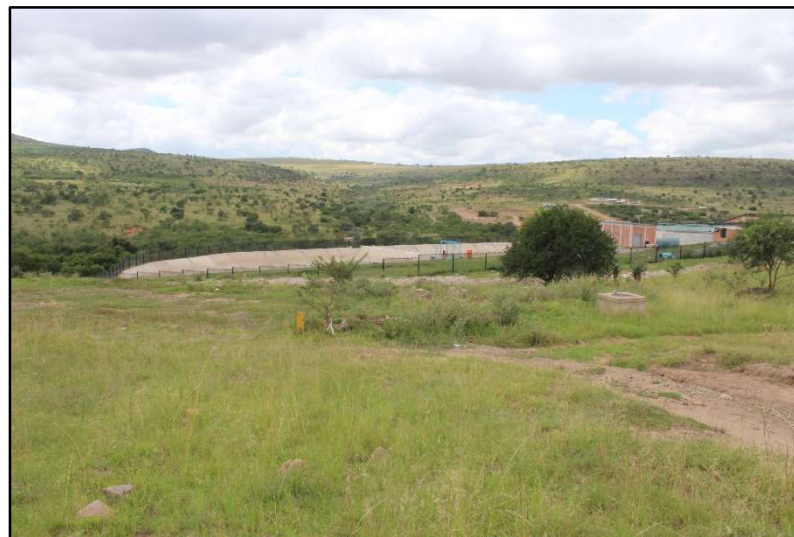
Plate 4: General view of the Cluster 9 Tsomo WTW Upgrade study site [4]
