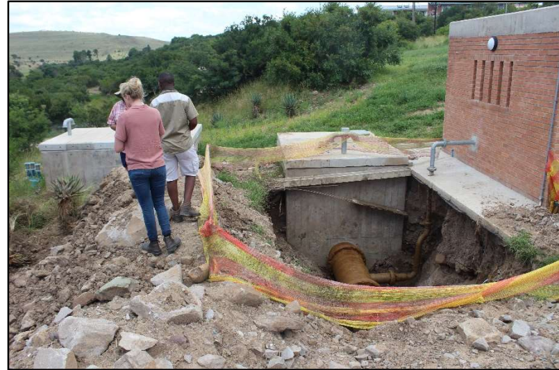
Plate 19: General view of the existing Tsomo WTW plant [3]
