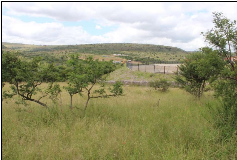
Plate 6: General view of the Cluster 9 Tsomo WTW Upgrade study site [6]
