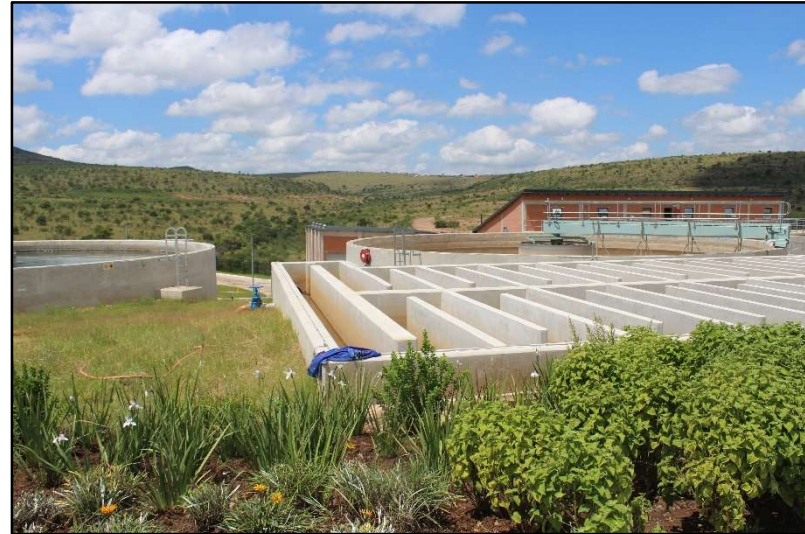
Plate 24: General view of the existing Tsomo WTW plant [6]
