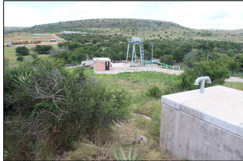
Plate 20: General view of the existing Tsomo WTW plant [4]
