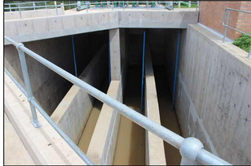
Plate 23: General view of the existing Tsomo WTW plant [5]
