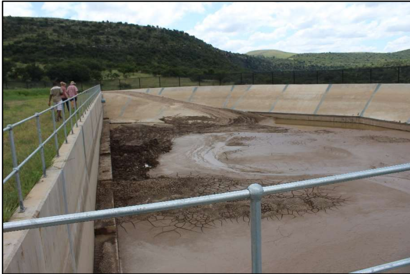
Plate 18: General view of the existing Tsomo WTW plant [2]
