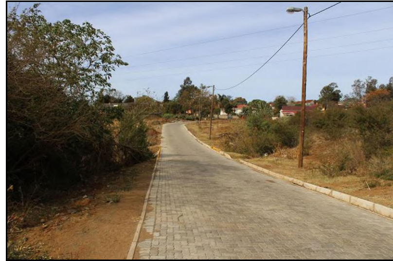
Plate 9: General view of the proposed line route development corridor [2]
