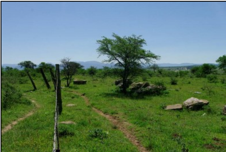
Plate 14: General view of Gravity Main 3 (from north to south) [2]
