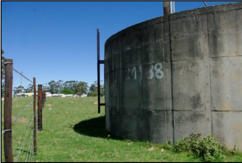
Plate 17: General view of the Gravity Main 4 (from north to south) [1]
