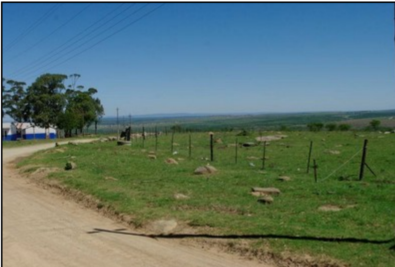
Plate 18: General view of the Gravity Main 4 (from north to south) [2]
