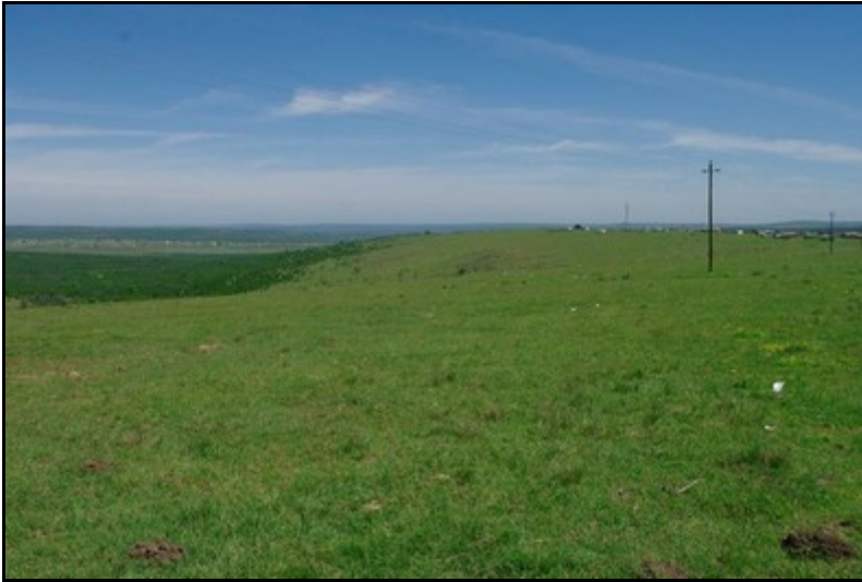
Plate 33: General view of the Rising Main 6 alignment [1]
