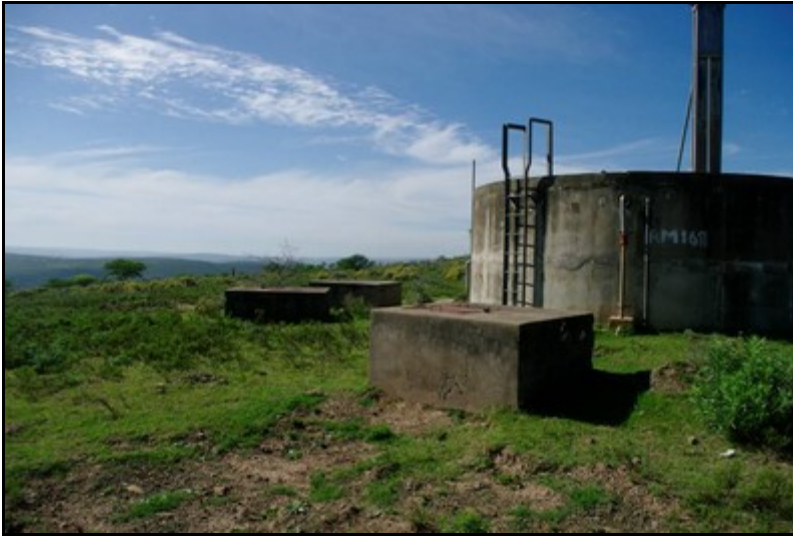
Plate 9: General view of Gravity Main 2 (from north to south) [1]
