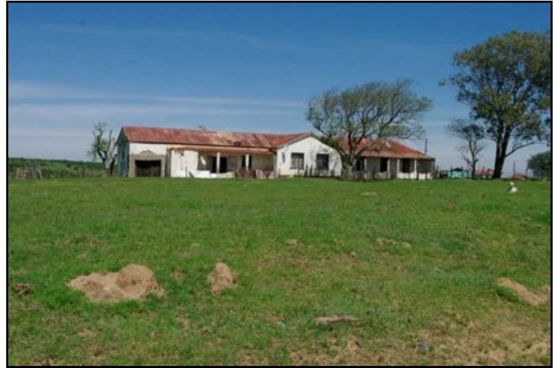
Plate 35: View of the Site D-RM6-S2 Colonial Period building
