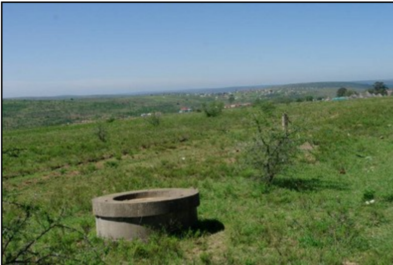
Plate 2: General view of the Gravity Main 1 alignment
