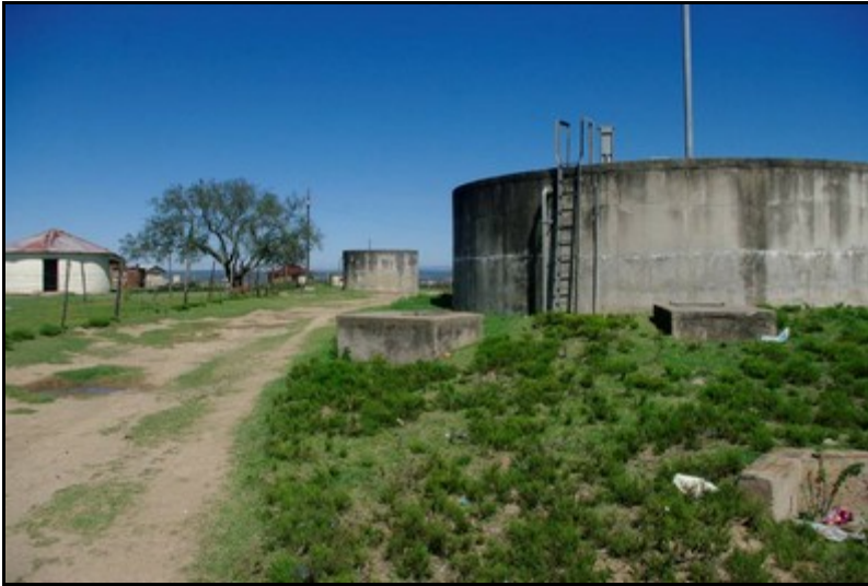
Plate 1: Beginning of the Gravity Main 1 alignment in Ncabasa Village
