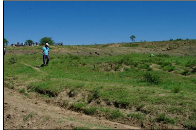
Plate 8: End of the Gravity Main 1 line route with Site D-GM1-S2 in the background
