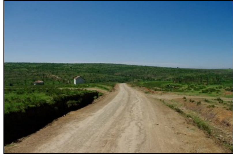
Plate 3: Gravity Main 1 alignment with Site D-GM1-S1 in the background
