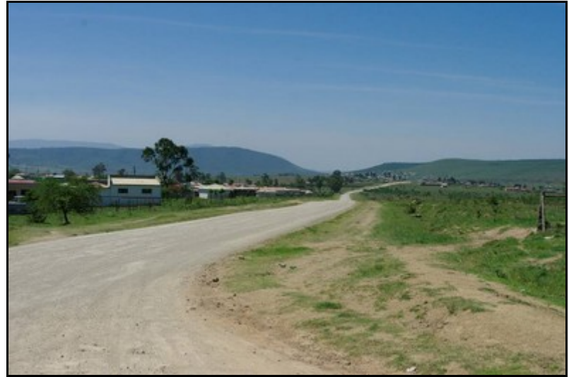
Plate 52: General view of the Gravity Main 8 alignment [2]
