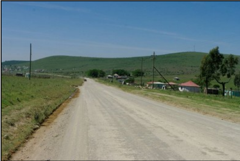
Plate 53: General view of the Gravity Main 8 alignment [3]
