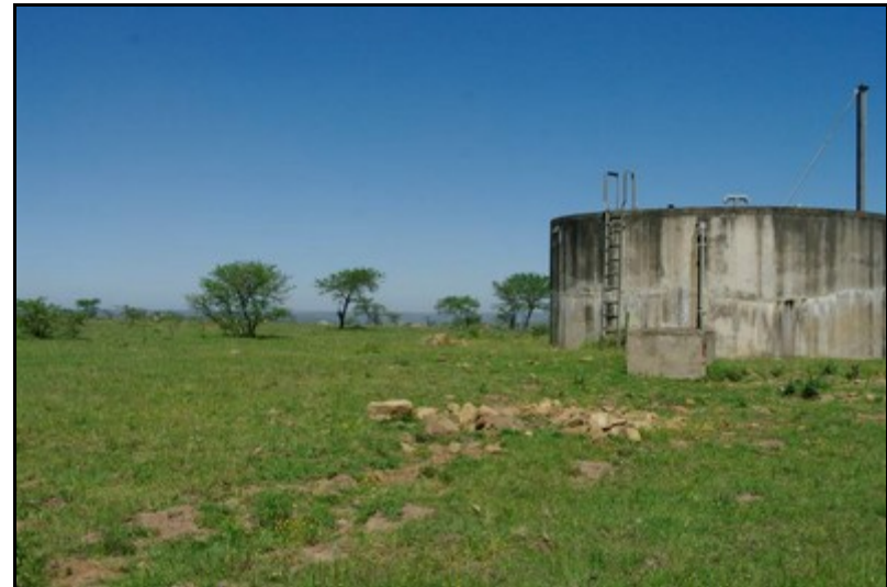
Plate 16: General view of Gravity Main 3 (from north to south) [4]
