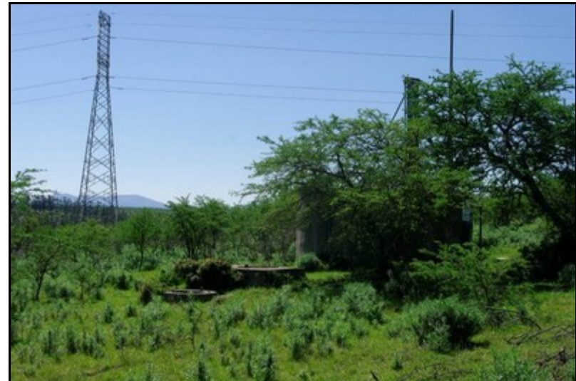
Plate 20: General view of the Gravity Main 4 (from north to south) [4]
