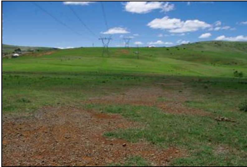
Plate 1: View of the Galatyeni substation SS-1 study site area
