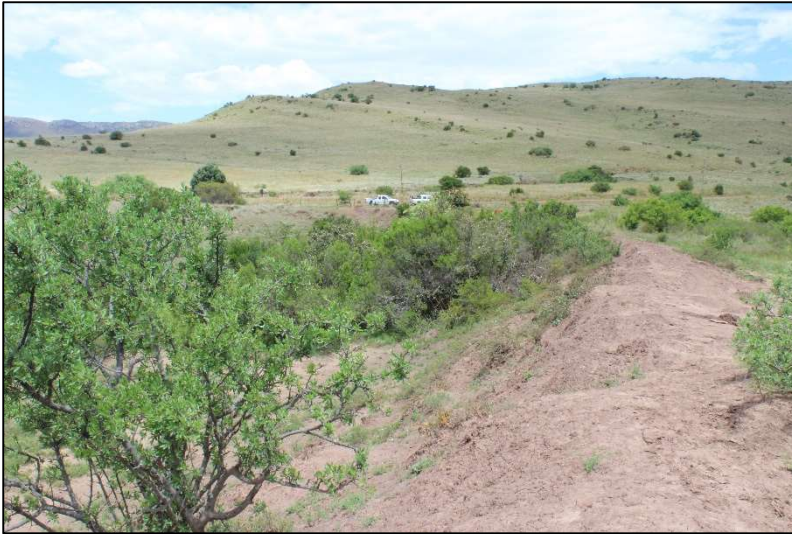
Plate 1: General view of the Helpmekaar Dam study site – dam wall [1]
