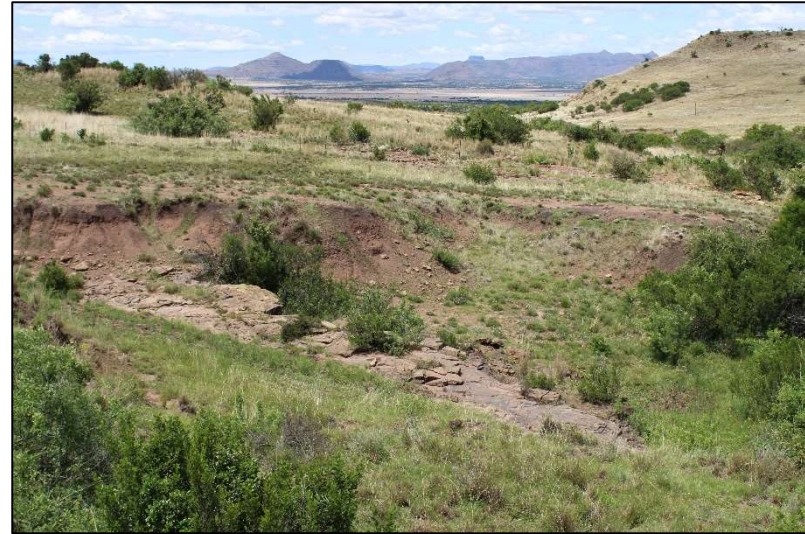
Plate 15: View from existing dam wall onto the spillway
