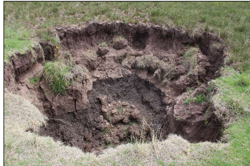
Plate 8: An eroded hole at the Helpmekaar Dam study site measuring approximately 1m in diameter
