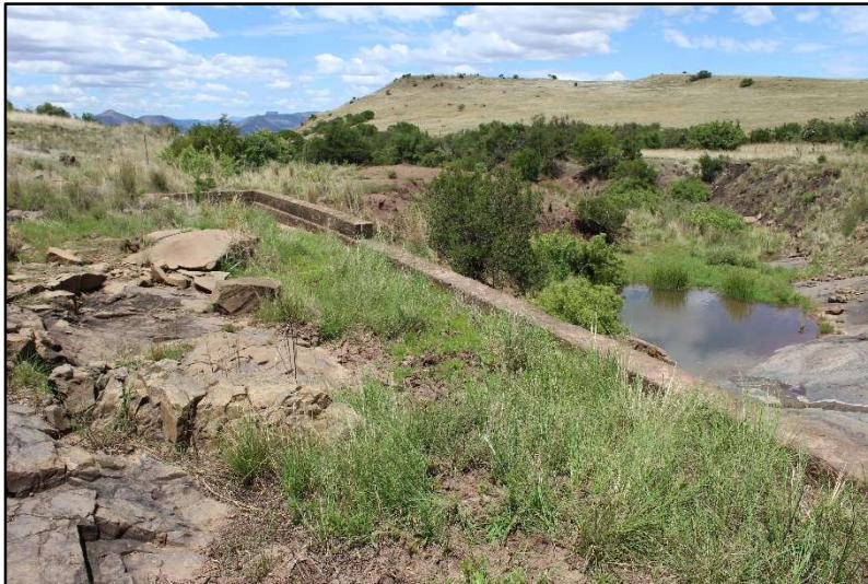
Plate 14: View from Site HN-02 onto the spillway
