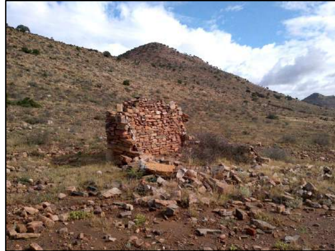
Plate 127: View of the stone structure 1 remains [1]
