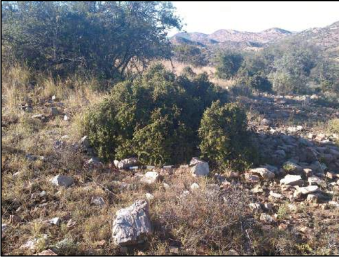
Plate 77: Circular stone foundation remains (1.5–2m in diameter) with a bush growing inside the structure
