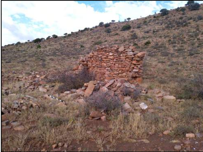
Plate 129: View of the stone structure 1 remains [3]
