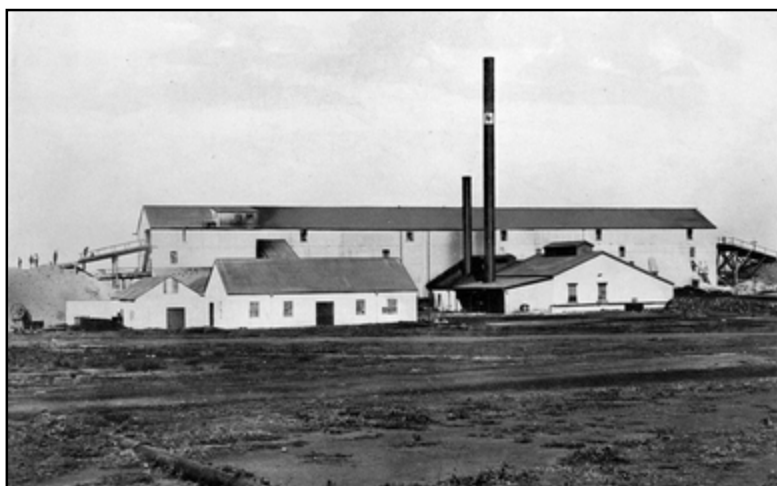
Plate 2: 'The Simmer & Jack Gold Mining Co. Ltd' plant, Elandsfontein, 1895 ( de.wikipedia.org/wiki/Simmer_and_Jack )
