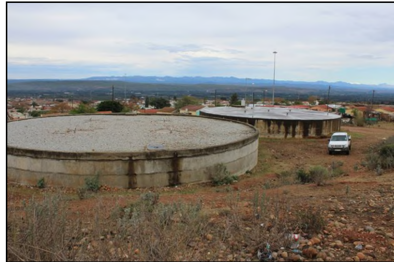
Plate 16: Existing Moses Mabida reservoir development
