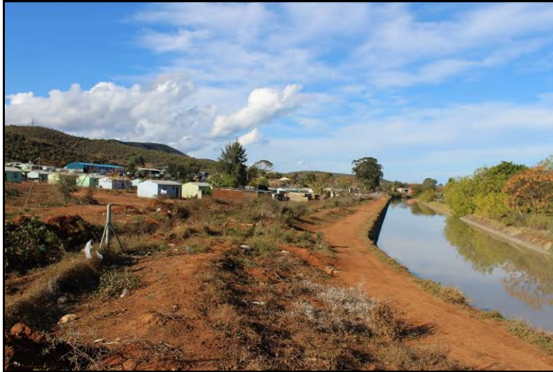
Plate 9: General view of the line route [8]
