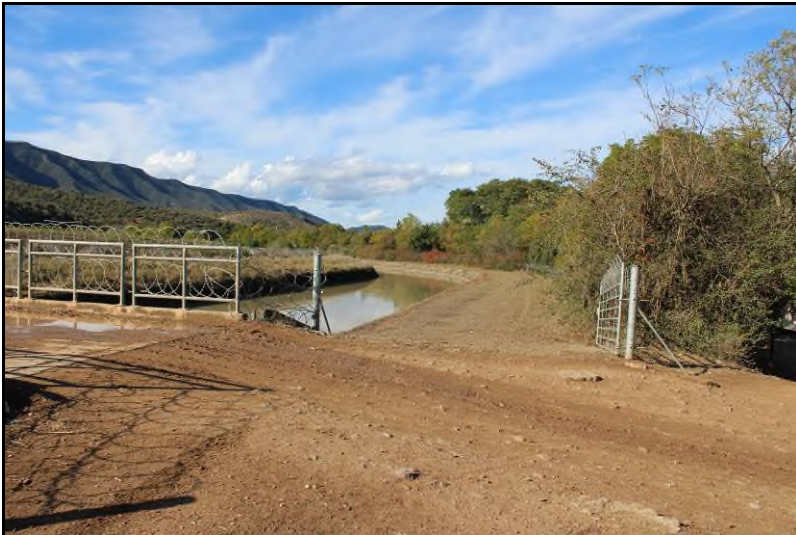
Plate 6: General view of the line route [5]
