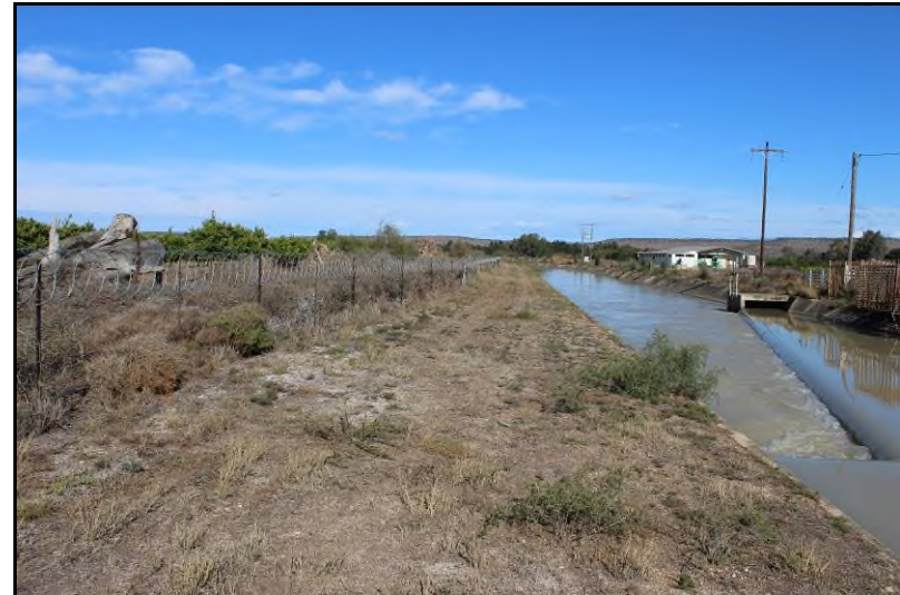
Plate 4: General view of the line route [3]
