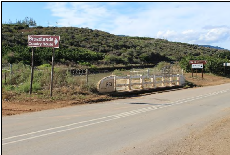
Plate 22: View of Site KBW-S2, the 1963 bridge across the canal
