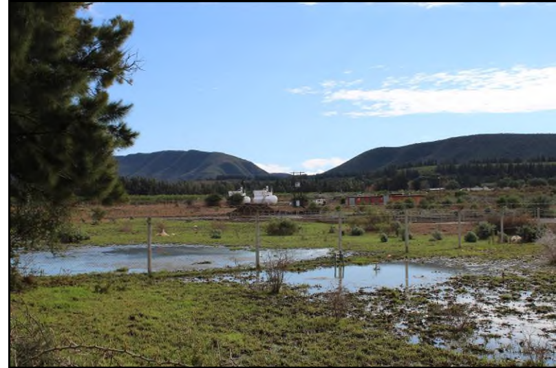
Plate 19: General view of the Kirkwood WWTW, Bontrug [1]
