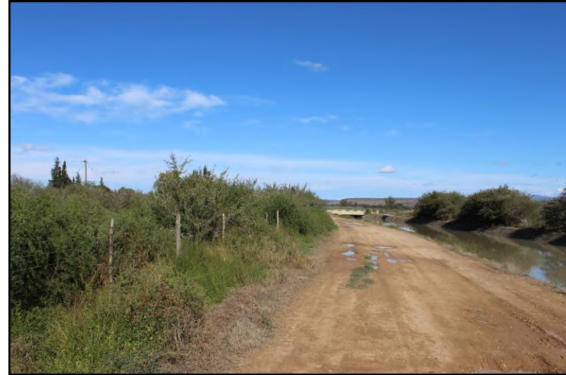
Plate 3: General view of the line route [2]
