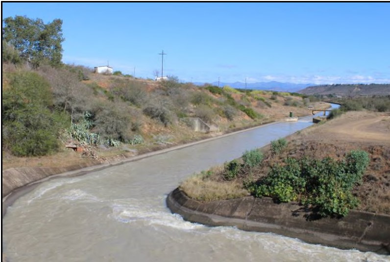
Plate 2: General view of the line route [1]
