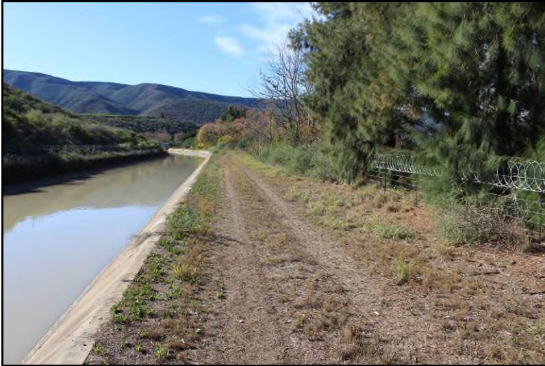
Plate 5: General view of the line route [4]
