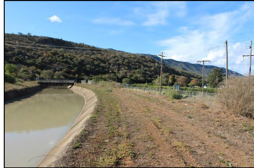
Plate 7: General view of the line route [6]
