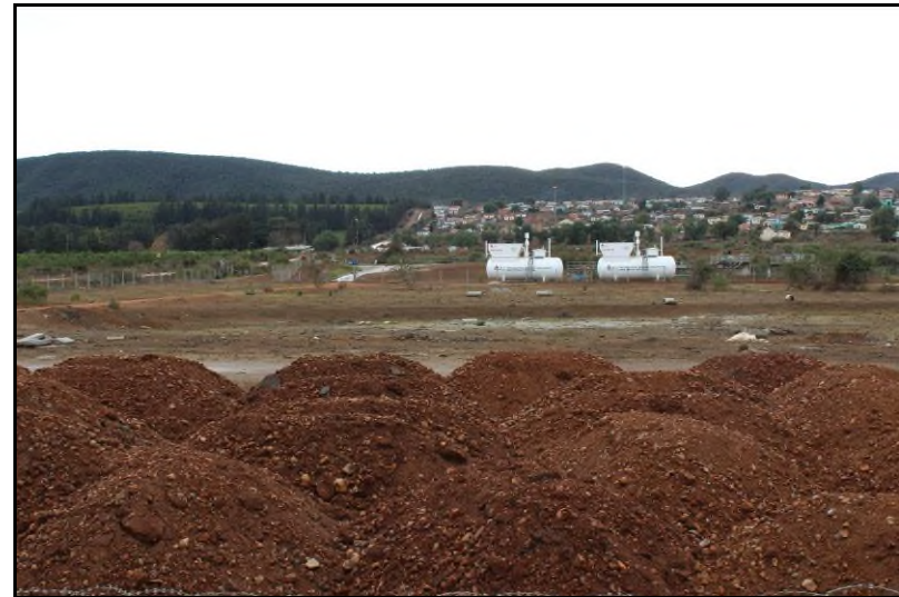
Plate 20: General view of the Kirkwood WWTW, Bontrug [2]
