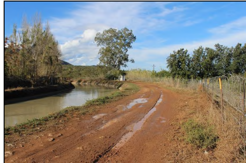
Plate 8: General view of the line route [7]
