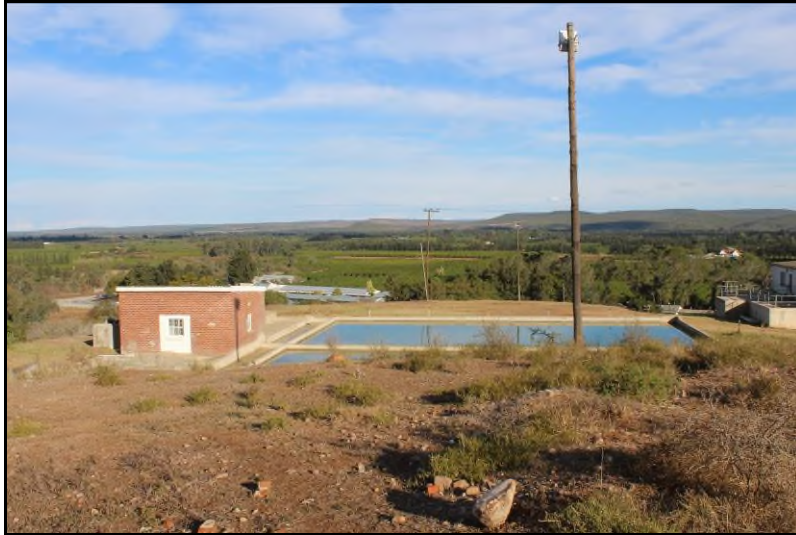
Plate 13: The Kirkwood WTW, with the proposed study site immediately adjoining the back pond
