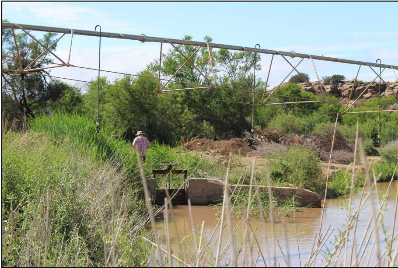
Plate 29: General view of the existing inlet
