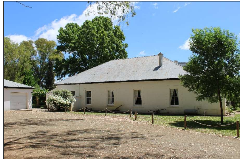
Plate 4: General view of Site LDS-01 [4]
