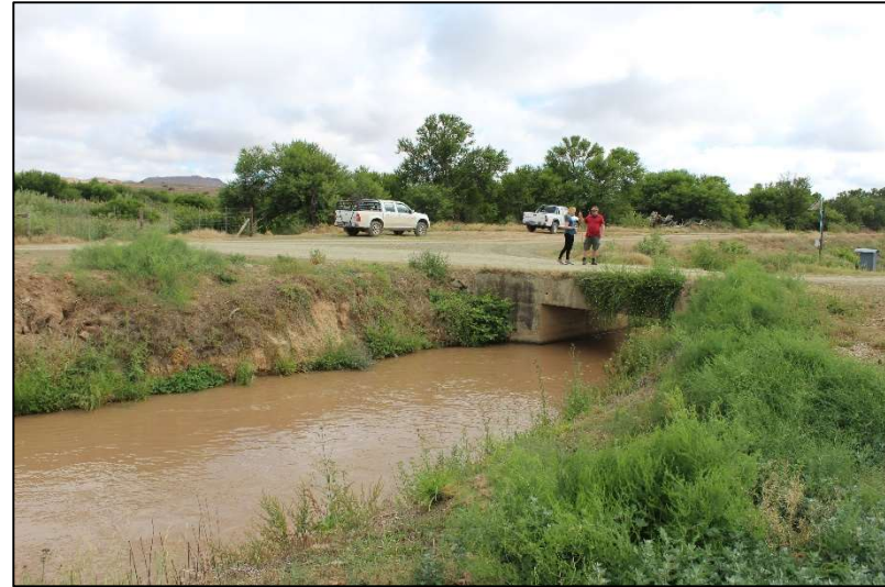
Plate 23: View across the canal near the weir with the measuring structure in the background
