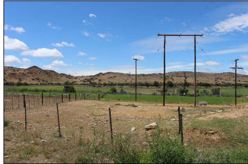
Plate 19: General view of the powerline route [3]
