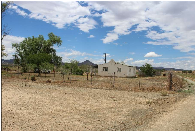
Plate 6: General view of Site LDS-02 [2]
