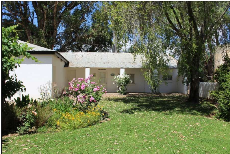
Plate 2: General view of Site LDS-01 [2]
