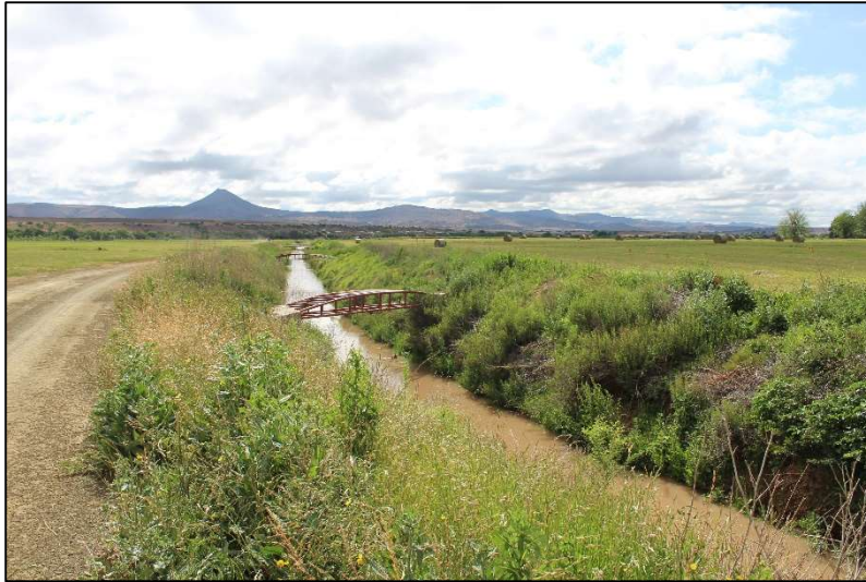
Plate 25: General view of the canal [2]
