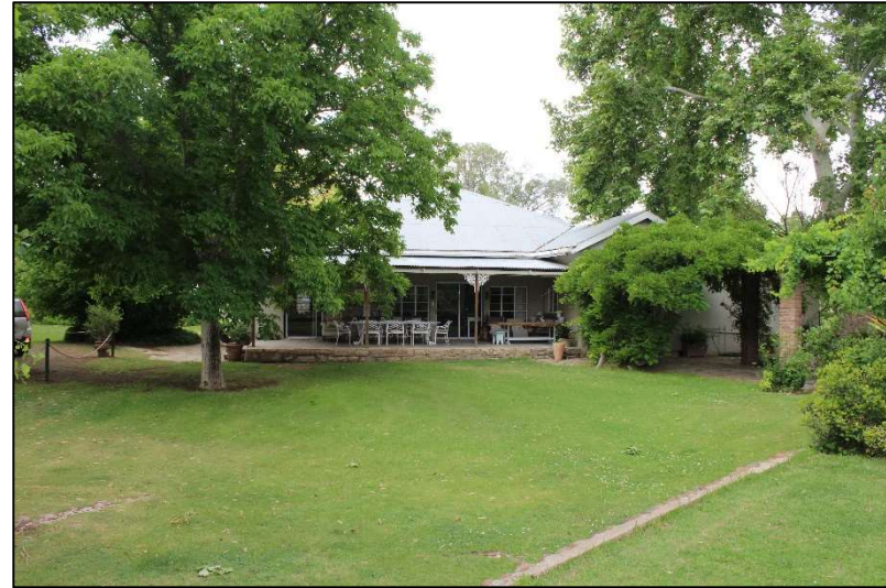
Plate 15: General view of Site LDS-04 [1]
