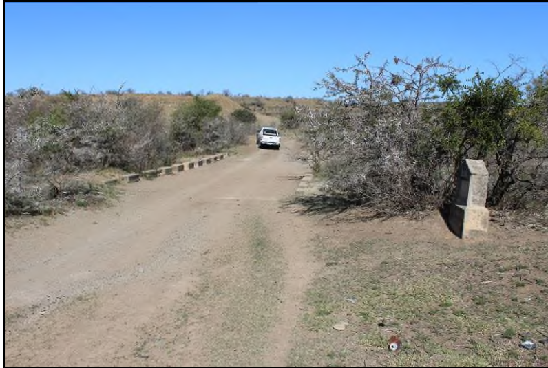
Plate 8: View of the Site FBA-S1 Colonial Period bridge [2]
