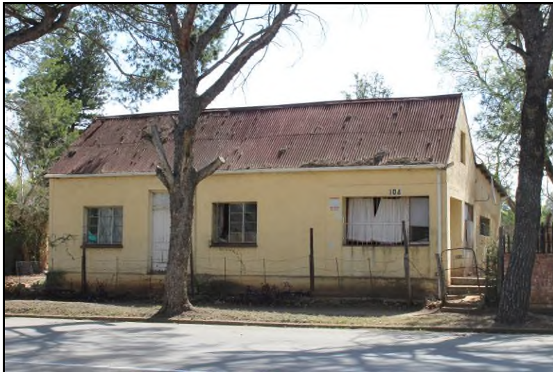
Plate 37: View of the Site FBA-S11 Colonial Period residence
