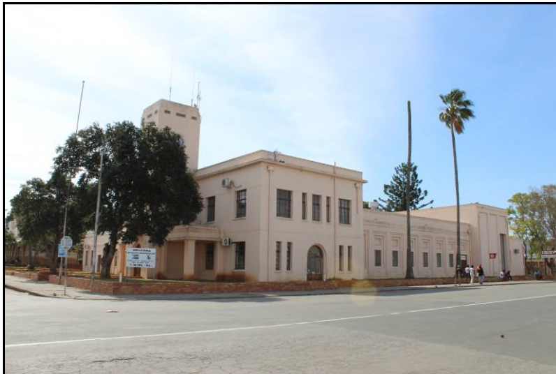
Plate 57: Site FBA-S32, the Colonial Period building used for municipal purposes [2]
