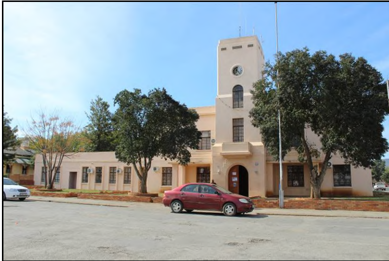
Plate 56: Site FBA-S32, the Colonial Period building used for municipal purposes [1]
