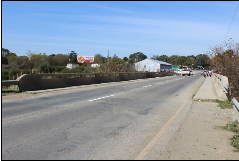
Plate 28: Bridge B4301 across the Kat River (near Site FBA-S4)
