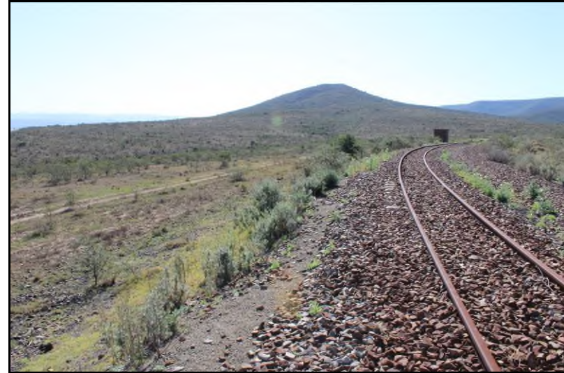
Plate 10: General view of the BP-07 study site from the railway line
