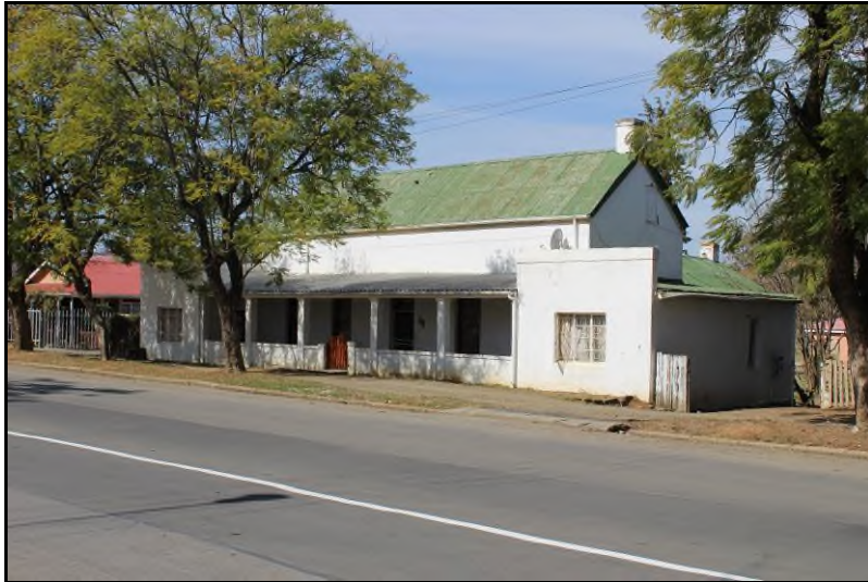
Plate 40: General view of the Site FBA-S14 Colonial Period residence
