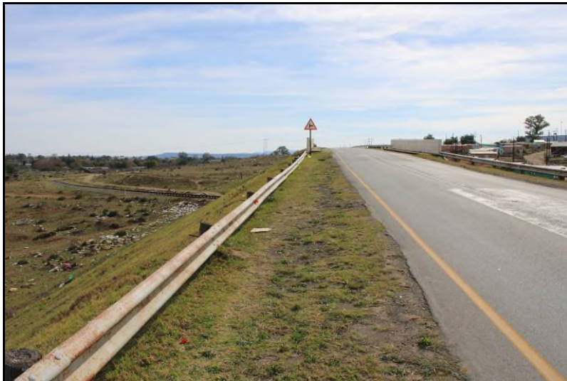
Plate 77: View of the Site FBA-S48 rail bridge
