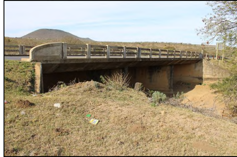
Plate 82: Site FBA-S51: General view of the Mxelo River bridge
