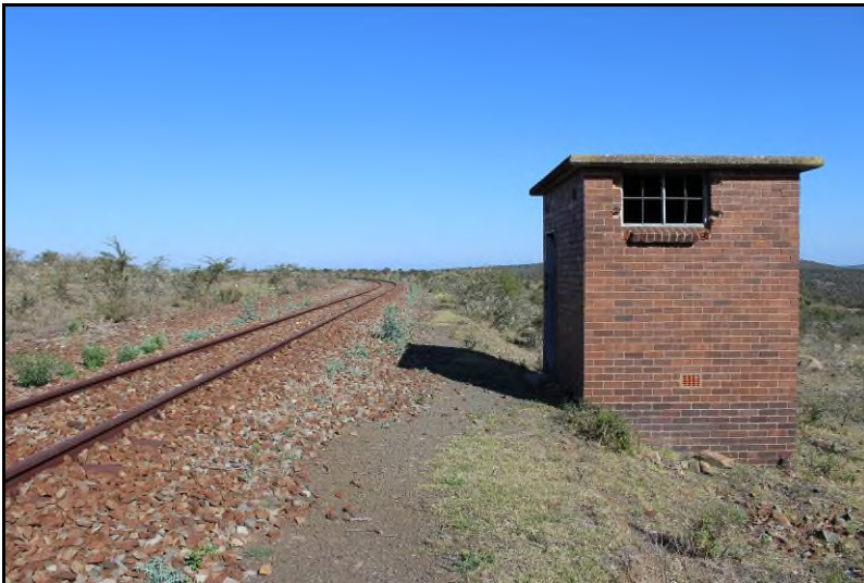
Plate 13: View of the Site FBA-S2 Colonial Period railway structure and line
