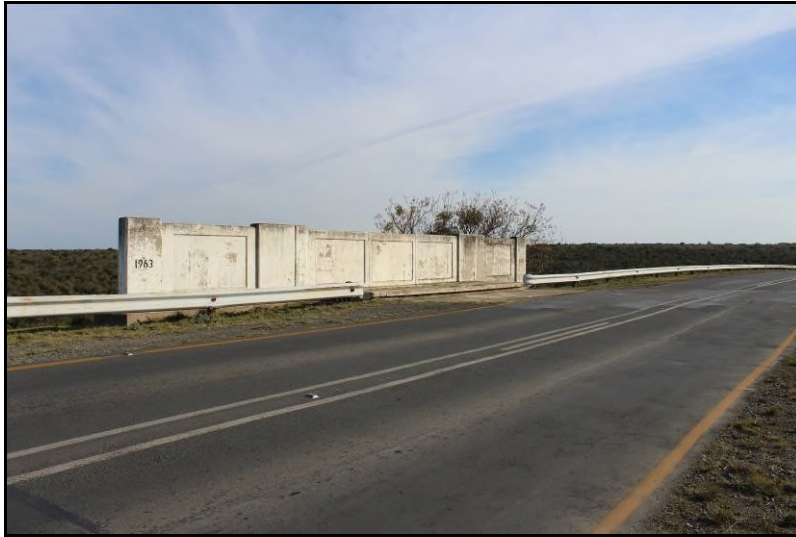
Plate 84: General view of the Site FBA-S53 rail bridge [1]
