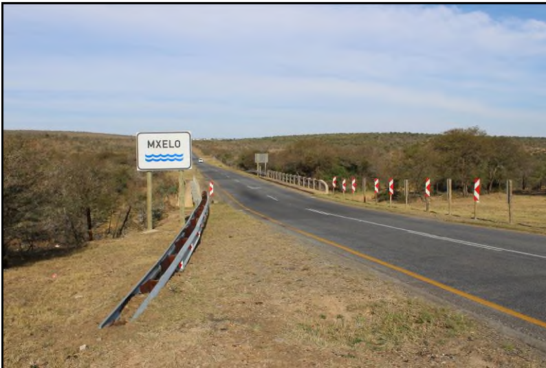
Plate 81: Site FBA-S51: View of the bridge across the Mxelo River
