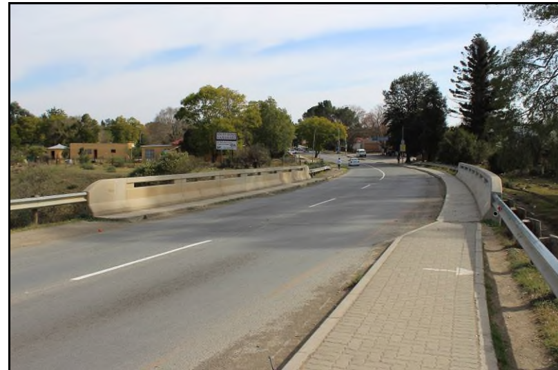
Plate 71: Site FBA-S46 – Contemporary bridge across the Kat River
