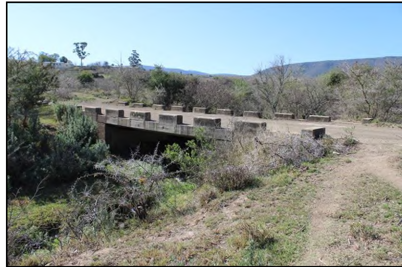
Plate 7: View of the Site FBA-S1 Colonial Period bridge [1]
