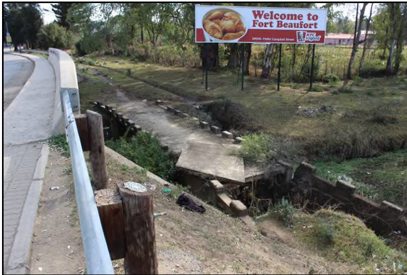
Plate 72: Site FBA-S46 – Colonial Period bridge across the Kat River [1]
