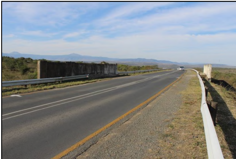
Plate 85: General view of the Site FBA-S53 rail bridge [1]
