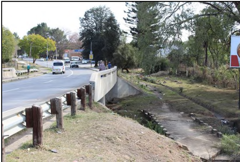
Plate 73: Site FBA-S46 – Colonial Period bridge across the Kat River [2]
