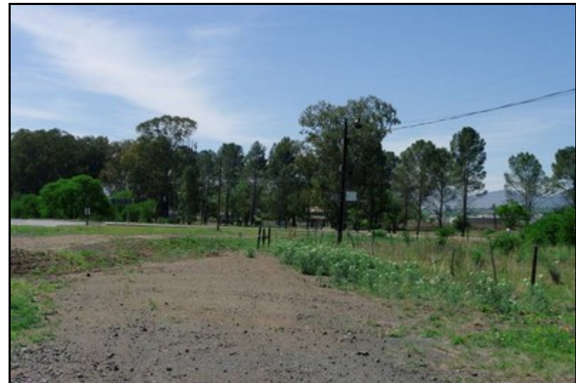
Plate 8: View of the effluent pipeline alignment with the Lukhanji WWTW across the R67
