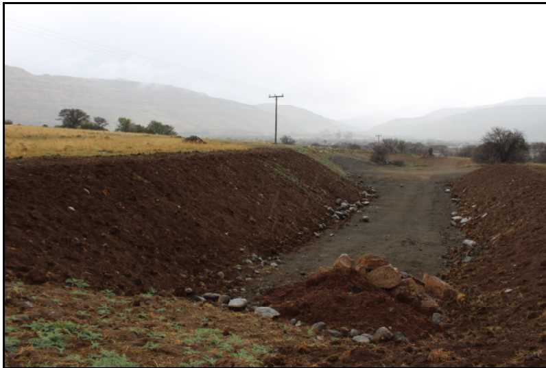
Plate 2: Current excavations and rehabilitation at the BP-01 study site
