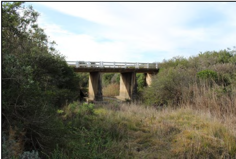
Plate 22: Site MR450-S7, the Coega River bridge [3]
