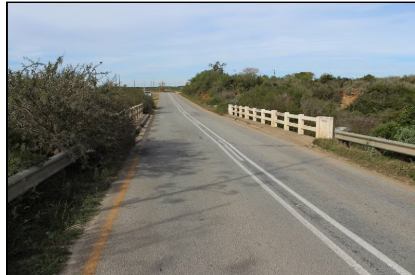
Plate 20: Site MR450-S7, the Coega River bridge [1]
