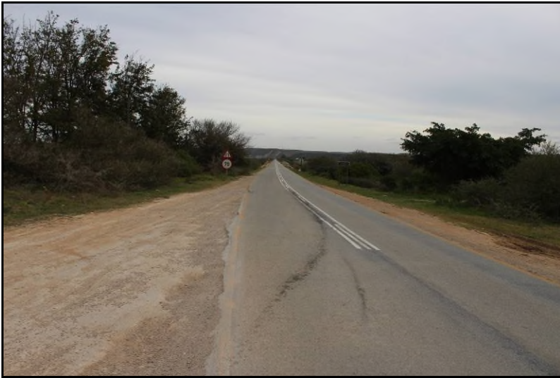
Plate 1: General view of the MR450 line route from its northern end, Addo
