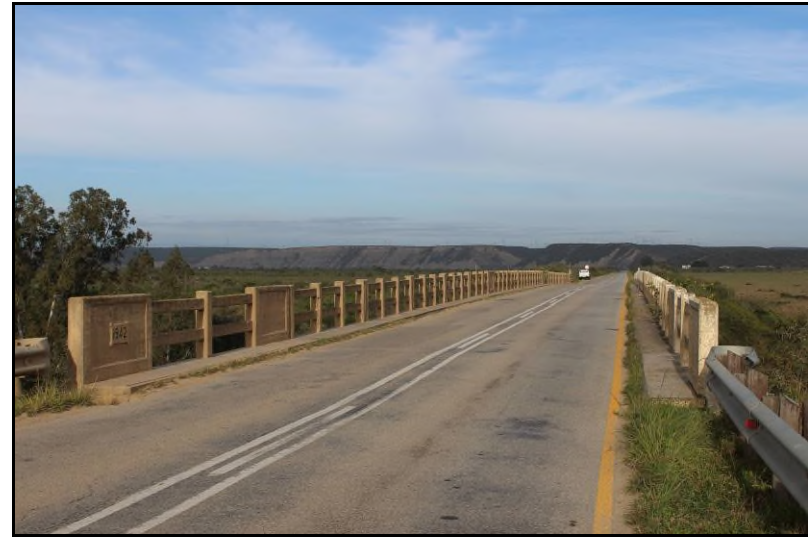
Plate 3: Site MR450-S1, the Sundays River bridge [2]
