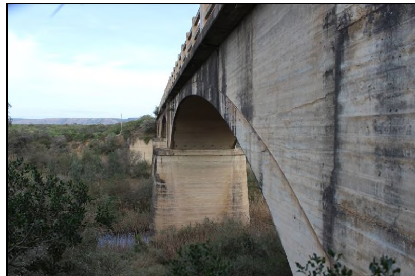
Plate 4: Site MR450-S1, the Sundays River bridge [3]
