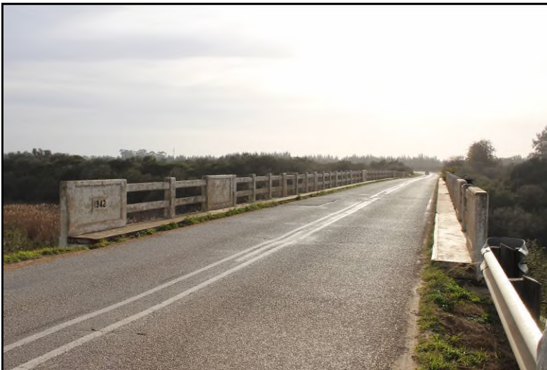
Plate 2: Site MR450-S1, the Sundays River bridge [1]
