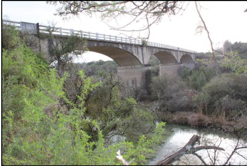
Plate 5: Site MR450-S1, the Sundays River bridge [4]
