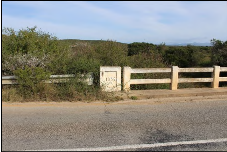
Plate 21: Site MR450-S7, the Coega River bridge [2]
