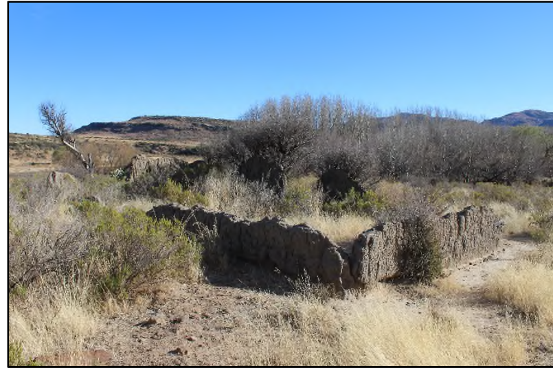
Plate 7: General view of 'The Mill', Site ZVD-S3 [3]
