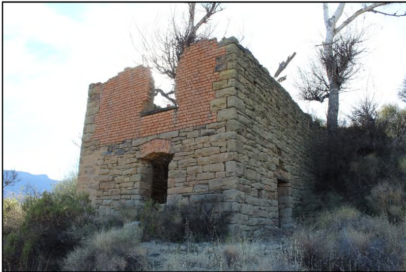
Plate 6: General view of 'The Mill', Site ZVD-S3 [2]
