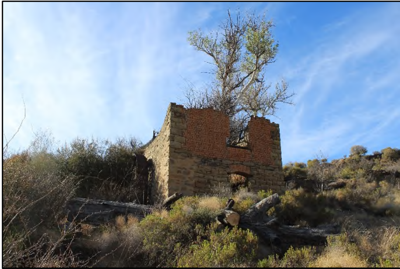
Plate 5: General view of 'The Mill', Site ZVD-S3 [2]
