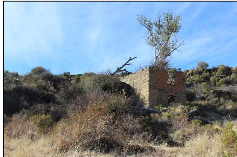
Plate 4: General view of 'The Mill', Site ZVD-S3 [1]
