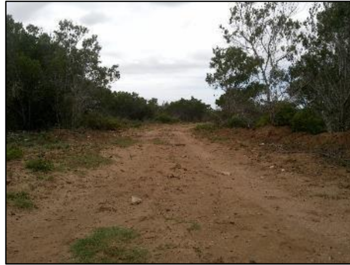
Plate 21: General view of access roads [1]
