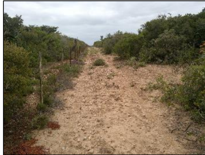
Plate 25: General view of access roads [5]
