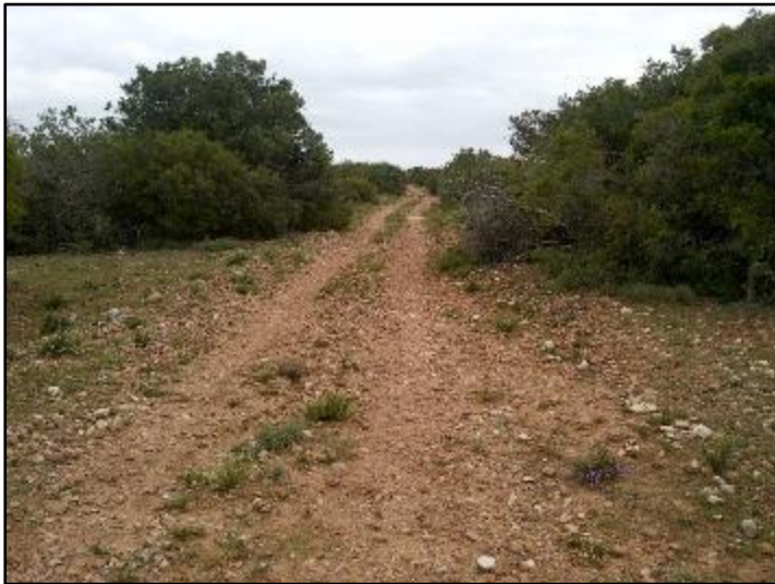
Plate 24: General view of access roads [4]
