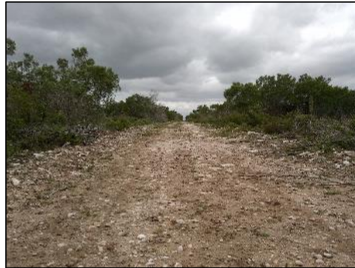
Plate 26: General view of access roads [6]
