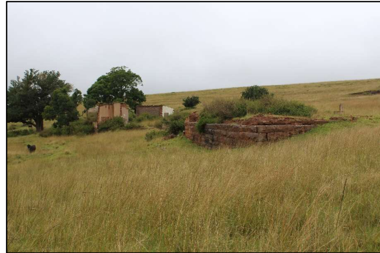
Plate 19: Structure remains at Site C9P5-02 [1]
