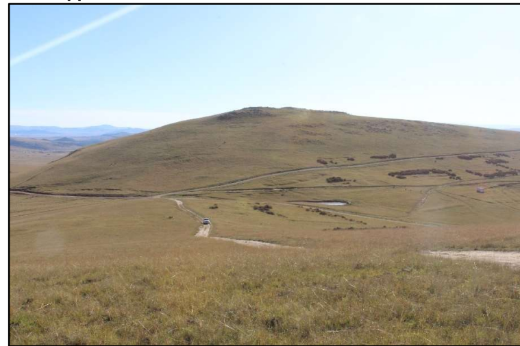
Plate 12: General view of the line route between the Nxamagele-Catshile link and the Catshile Reservoir [3]
