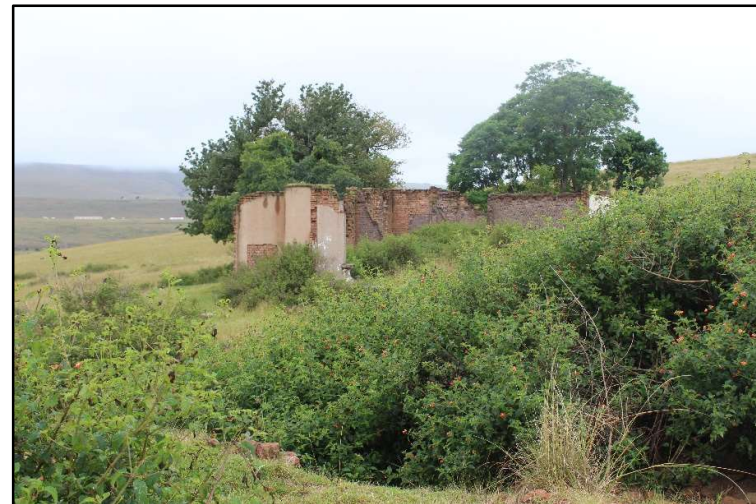
Plate 20: Structure remains at Site C9P5-02 [2]
