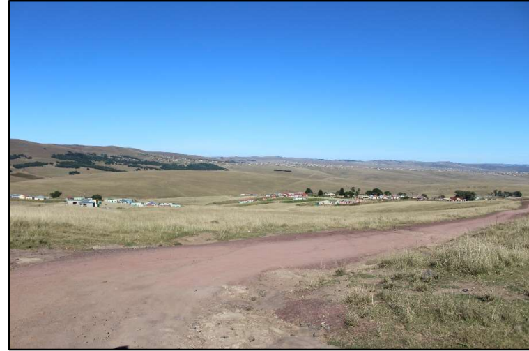
Plate 11: General view of the line route between the Nxamagele-Catshile link and the Catshile Reservoir [2]
