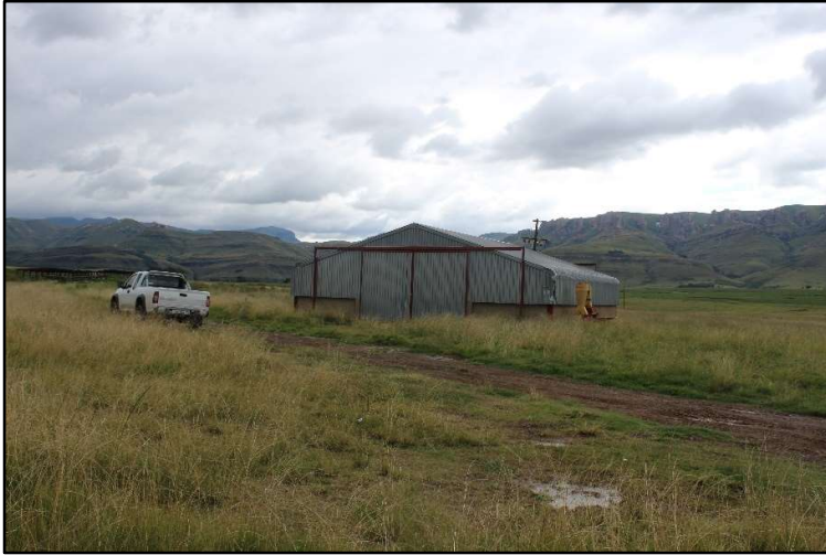
Plate 33: IFASS – View of the shed
