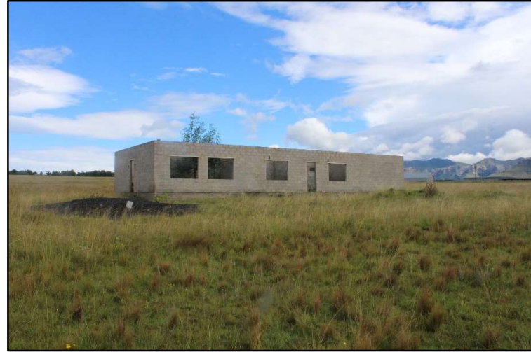
Plate 43: IFASS – The unfinished offices
