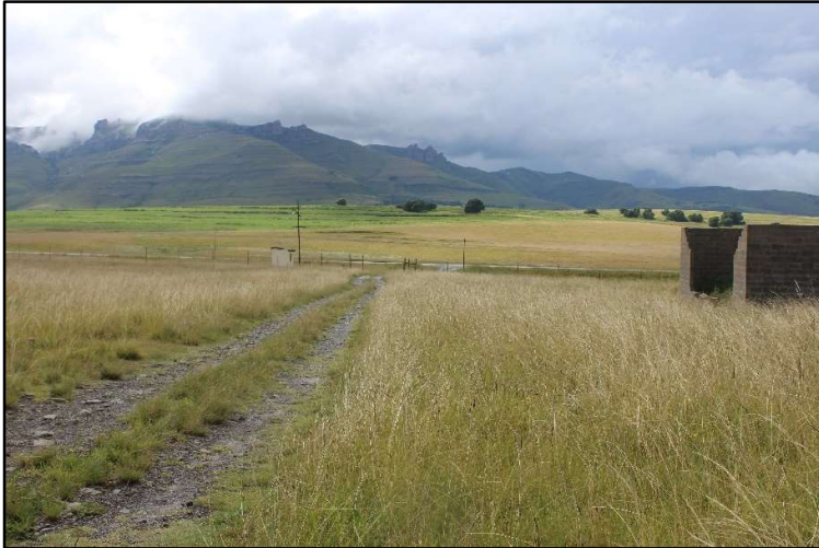
Plate 42: IFASS – Access road with the guard house in the background and unfinished offices
