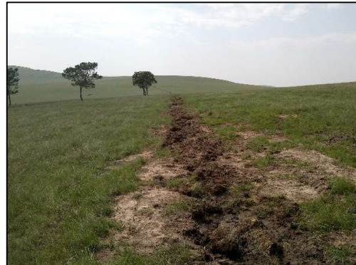
Plate 4: Accidental pipeline impact near Site C9P5-06
