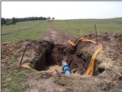
Plate 2: General view of the pipeline route at Sensitive Area 1 [2]
