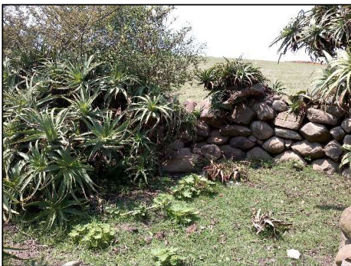
Plate 48: Close-up of stone kraal walls [2]
