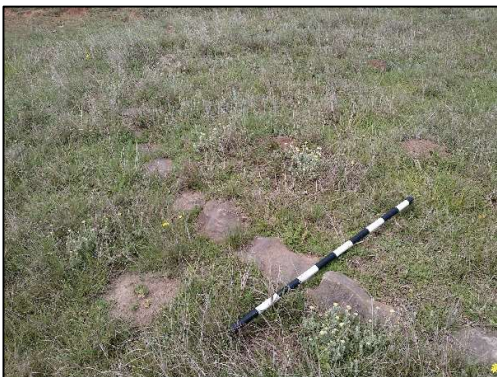
Plate 16: Close-up of hut foundations
