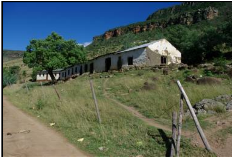
Figure 14: General view of Site BRME1
