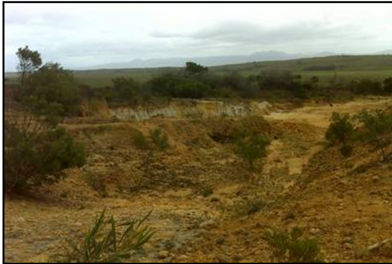
Figure 8: Current large scale impact at borrow pit 1763_BP02
