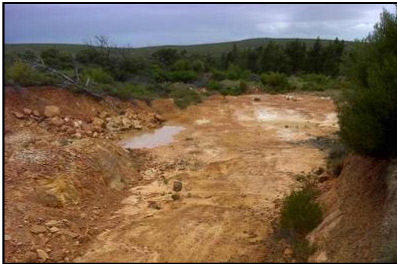
Figure 10: Current large scale impact at borrow pit 397_BP01
