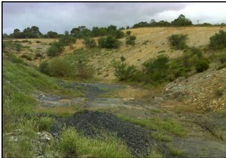
Figure 6: General view of borrow pit 1763_BP01
