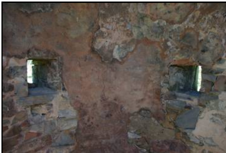
Figure 21: Close-up of defense slits in one of the tambours
