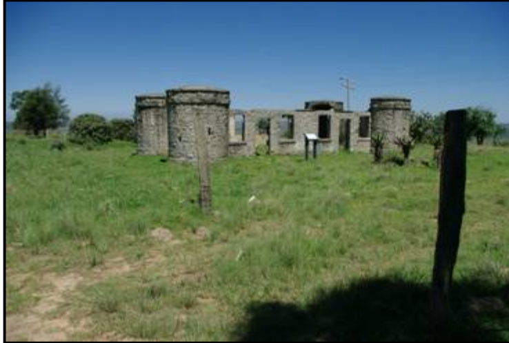
Figure 18: General view of the gangers' cottage with original conservation gate posts in the front
