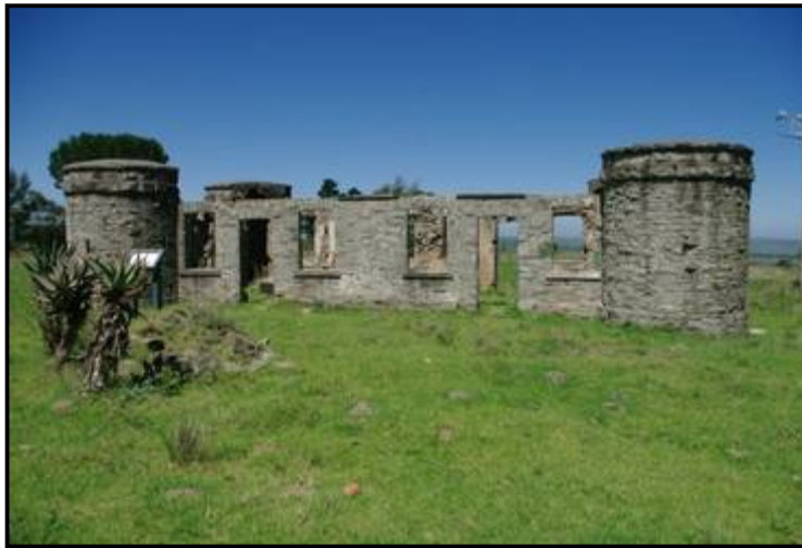
Figure 19: General view of the 'Fortified Gangers' Cottage No 17'
