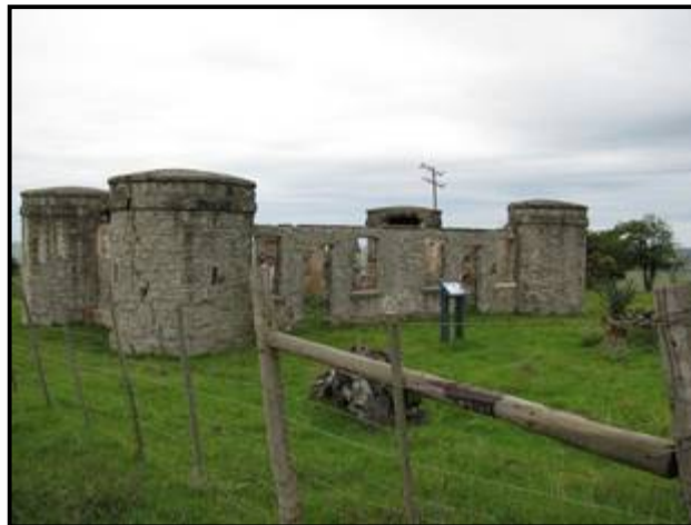
Figure 17: Fortified Gangers' Cottage No 17 (Dion T. – http://www.panoramic.com/photo/17711415 )
