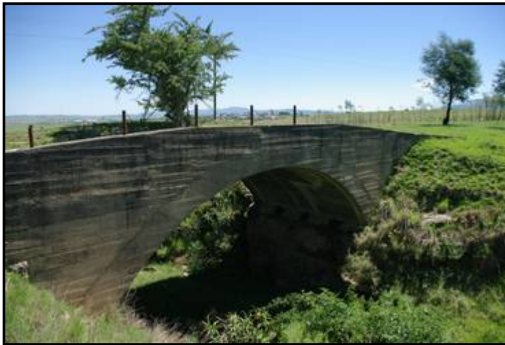
Figure 29: Close-up of the Railway Bridge – 1
