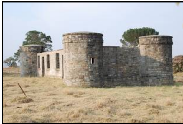
Figure 16: Fortified Gangers' Cottage No 17 (W. Martinson – http://www.artefacts.co.za/main/Buildings/10830 )
