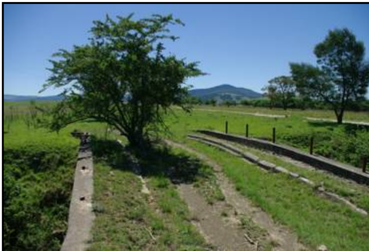
Figure 30: Close-up of the Railway Bridge – 2
