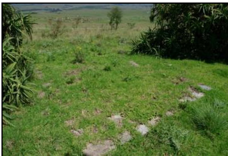
Figure 26: Foundation structure remains situated just south of F4
