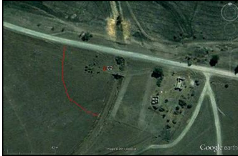
Figure 27: Site C2 – Railway Bridge
