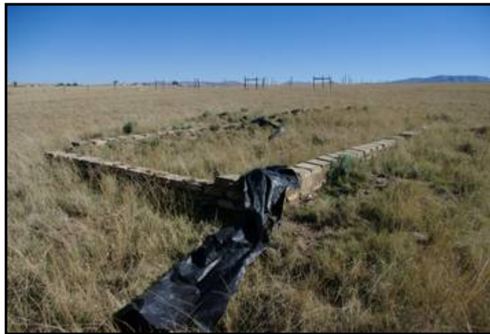
Figure 9: Contemporary structure foundations located within the generally assessed area around Qumanco
