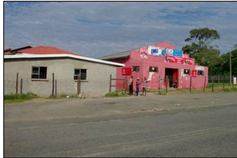
Plate 12: View of the SS7 contemporary structures
