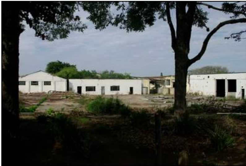
Plate 14: Contemporary structures at Ncera Macadamia Farming
