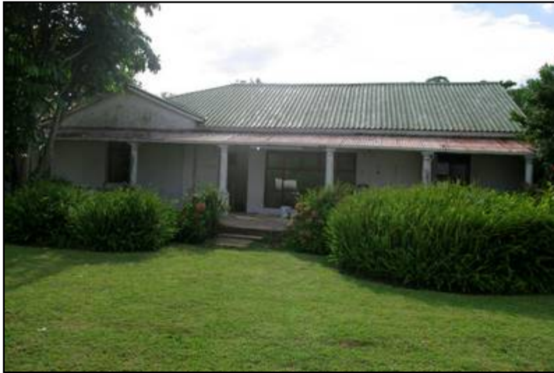
Plate 13: General view of the SS-3 Colonial Period residence
