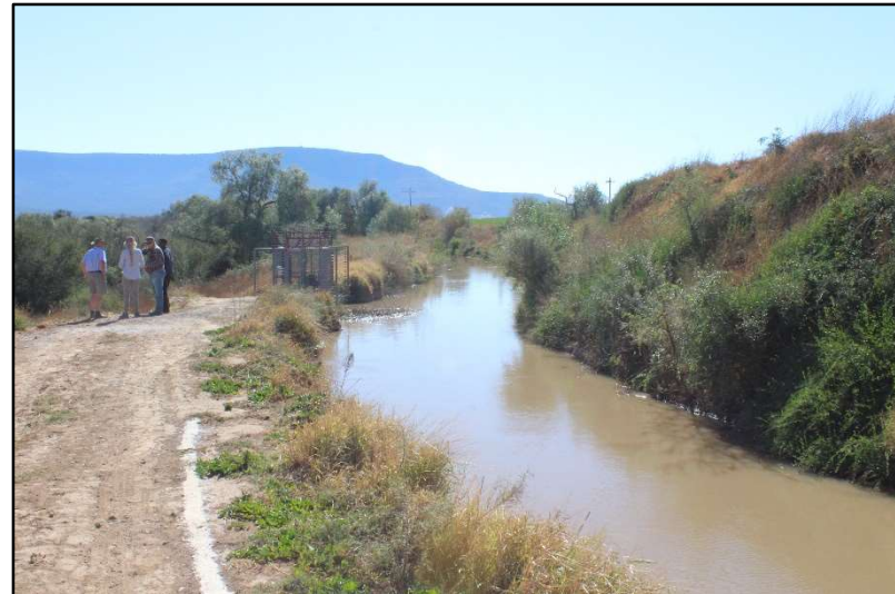
Plate 4: View of the existing pump station and outlet near Site BCD-01
