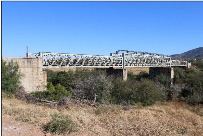
Plate 2: View of the Site BCD-01 railway bridge [2]
