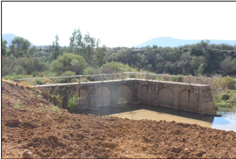
Plate 14: Existing infrastructure in the vicinity of the off-stream water storage dam [2]
