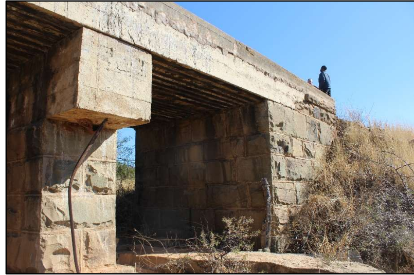
Plate 7: View of the Site BCD-02 railway bridge [2]
