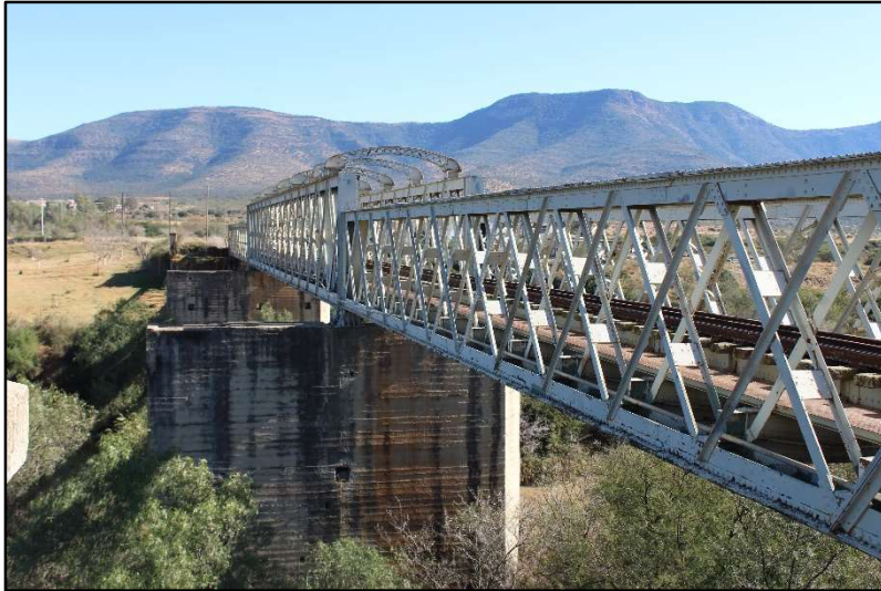
Plate 1: View of the Site BCD-01 railway bridge [1]
