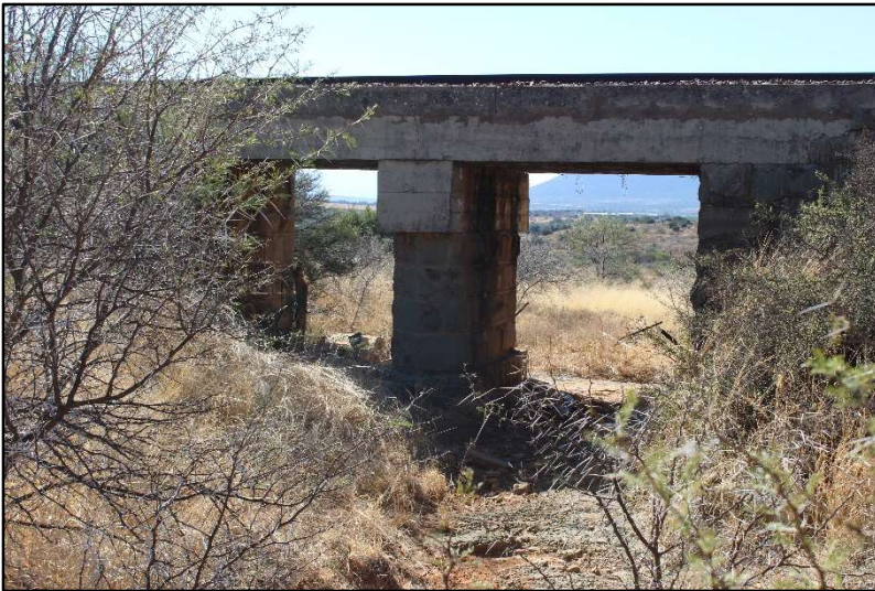
Plate 6: View of the Site BCD-02 railway bridge [1]
