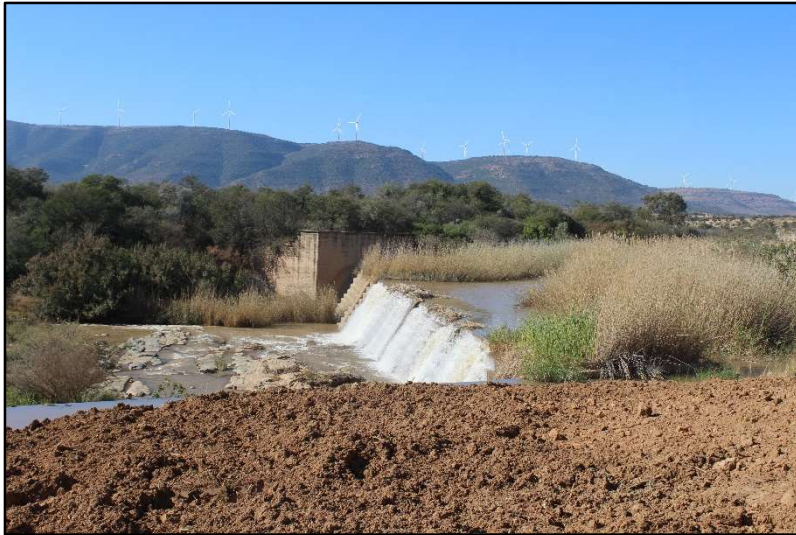
Plate 13: Existing infrastructure in the vicinity of the off-stream water storage dam [1]
