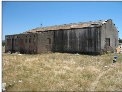
Figure 11. Back of the building
