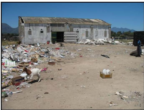
Figure 10. Metal and concrete building
