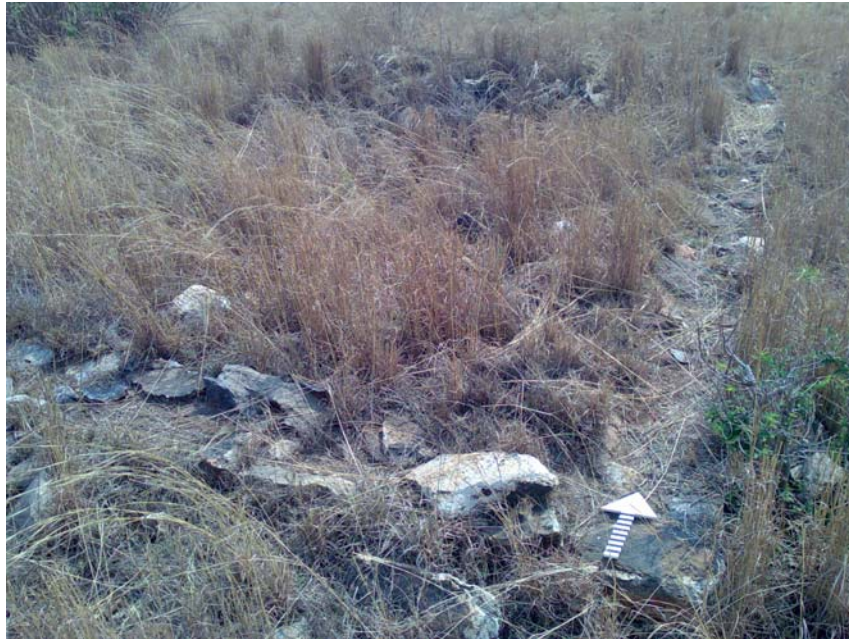
Figure 7: Stone foundation of the house.
