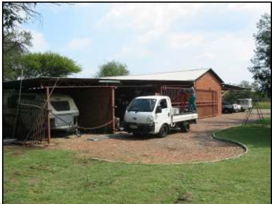
• Figure 4: Modern outbuildings on holding 124
