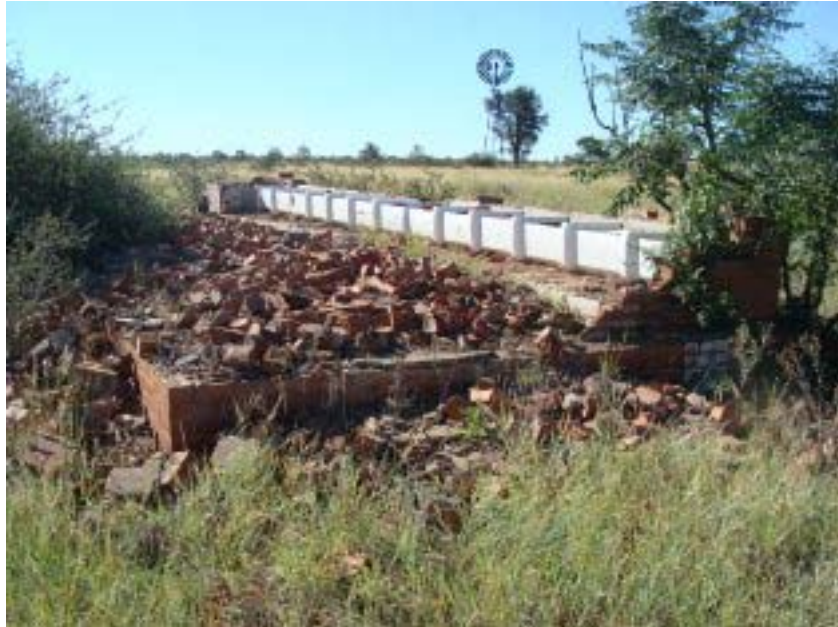
Figure 11: Remains of bathroom facilities on the site.
