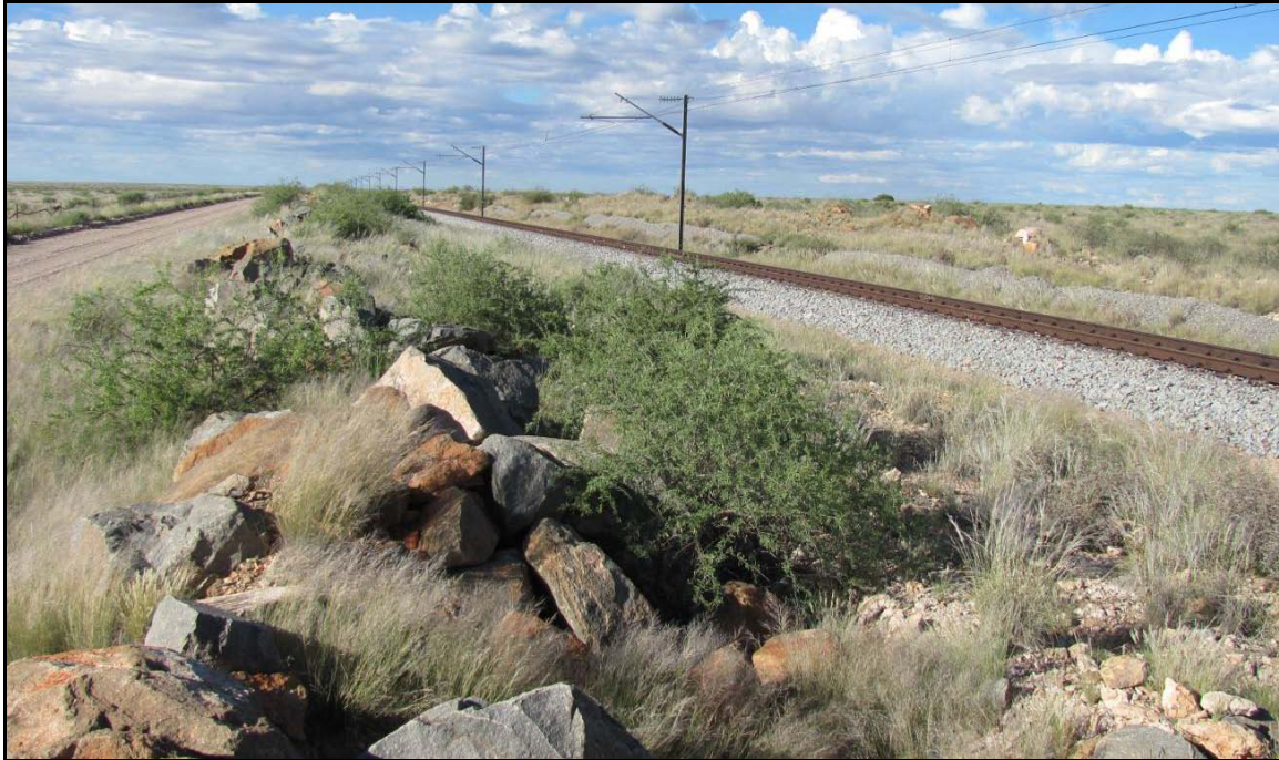
Plate 1: View of the railway line, the gravel service road and the large boulders which were uncovered during the construction of the line.
