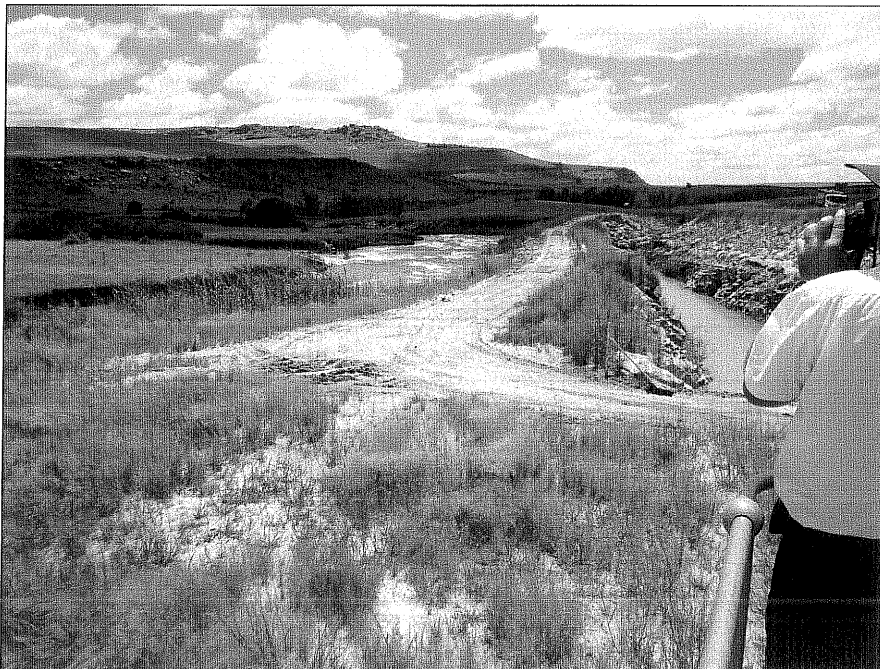
Fig.3 Water extraction channel (right) and the original flow of the Asrivier (left).
