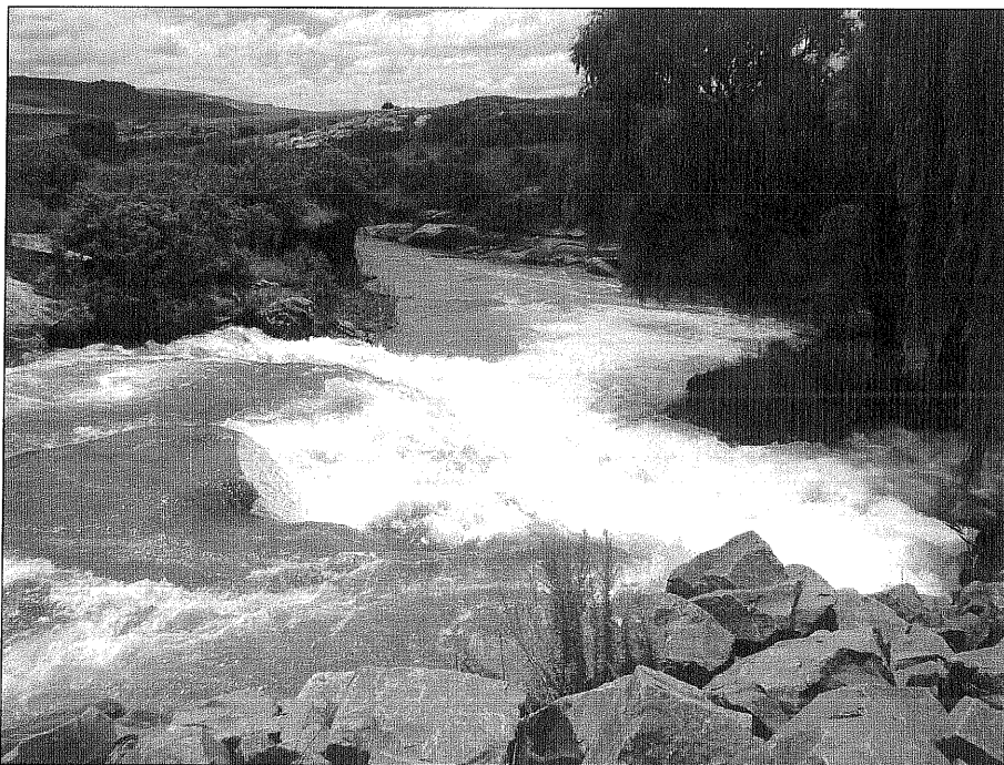
Fig.7 Proposed hydro-electric power plant site at Lower Kruisvallei 190.
