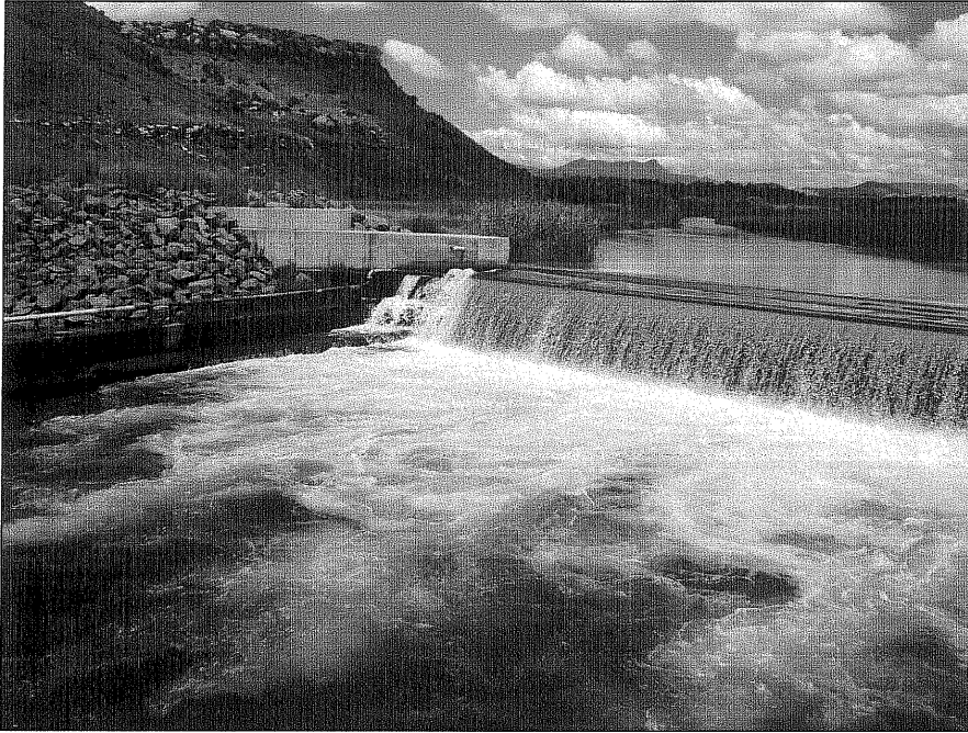
Fig.10 Water extraction weir at hydro-electric power plant at Middle Kruisvallei 190.
