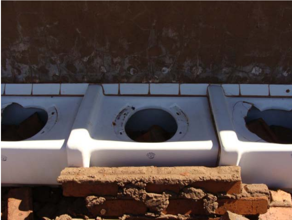
Figure 80 Part of the row of toilets inside of the building.
