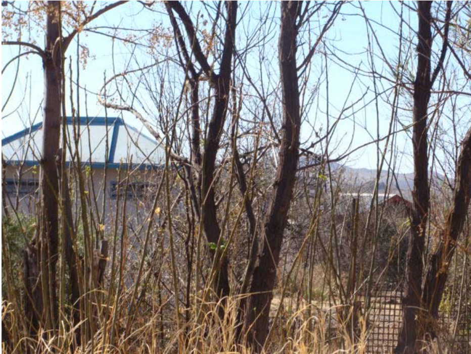
Figure 60 Pump house close to the village also from a more recent period.
