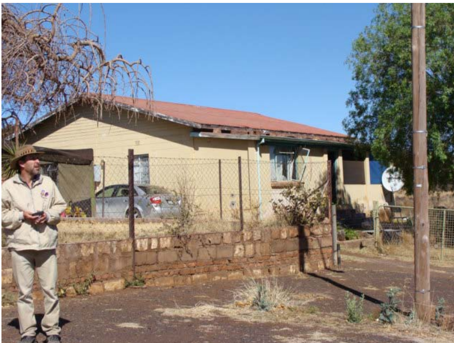
Figure 66 House number 3 at site number 4.
