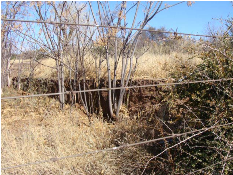
Figure 19 Stone structure, probable a water reservoir for the village.
