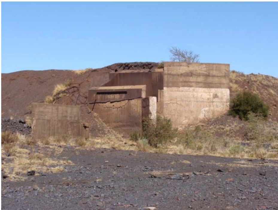
Figure 74 Remains of an ore loading bay.
