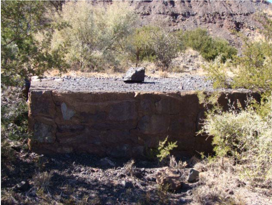
Figure 76 The loading platform.
