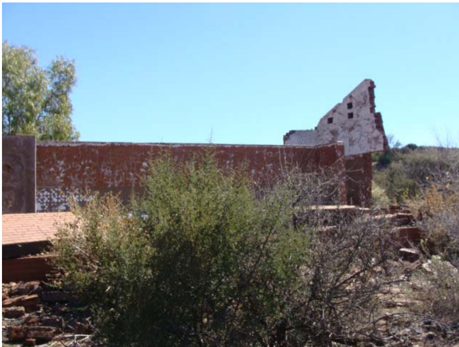
Figure 79 Remains of the toilet building.
