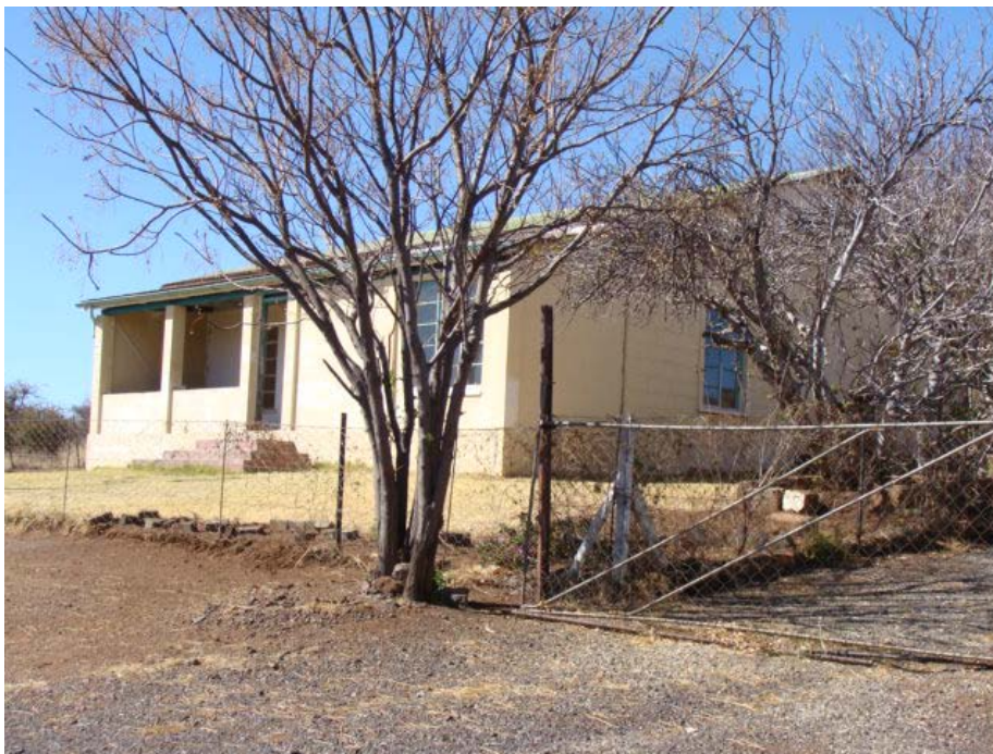
Figure 64 House number 1 at site number 4.
