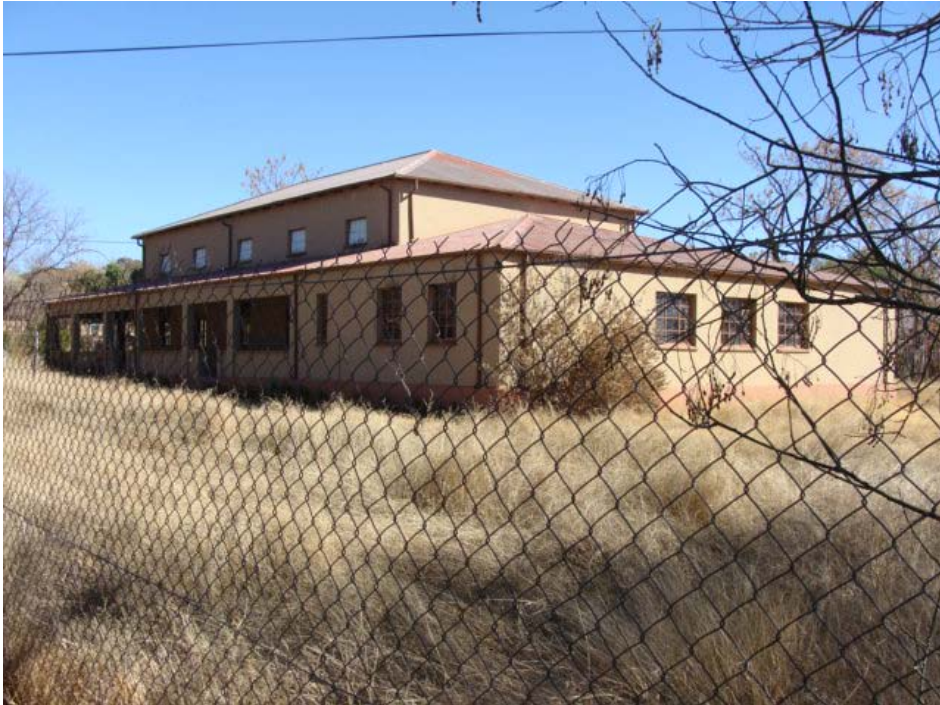
Figure 32 Back side of hall.
