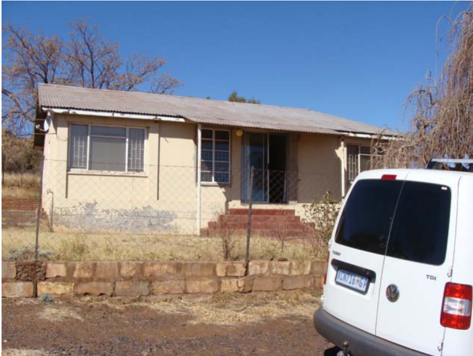
Figure 65 House number 2 at site number 4.
