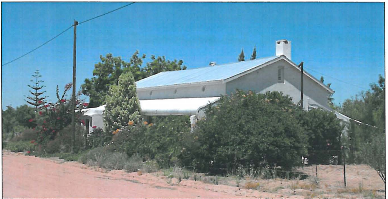
Plate 34: This house in Aurora may originally date to the late 19 th century.
