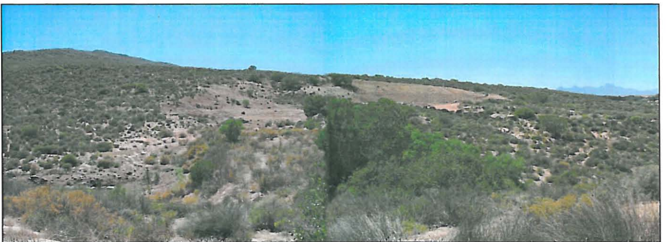
Plate 7: View towards the east over the existing borrow pit and the steep hillside to its north.
