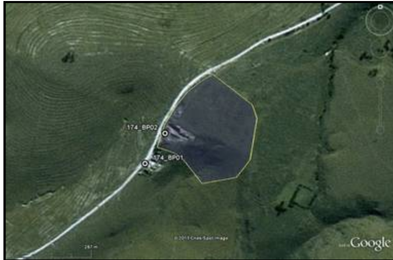
Figure 43: Borrow pit 174_BP02
