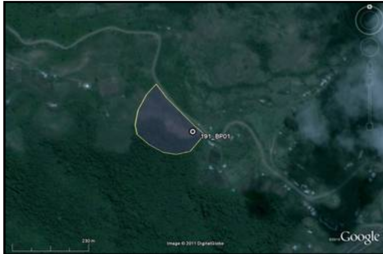
Figure 46: Borrow pit 191_BP01
