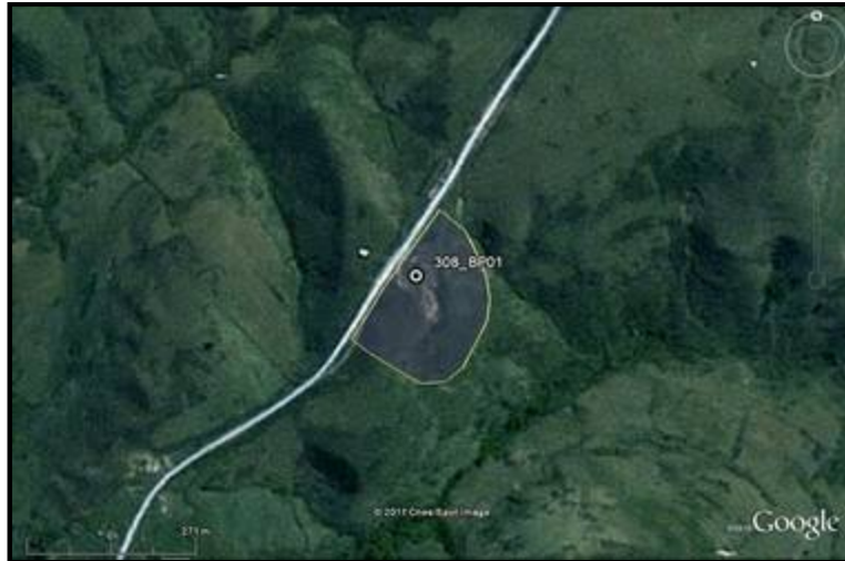
Figure 53: Borrow pit 308_BP01
