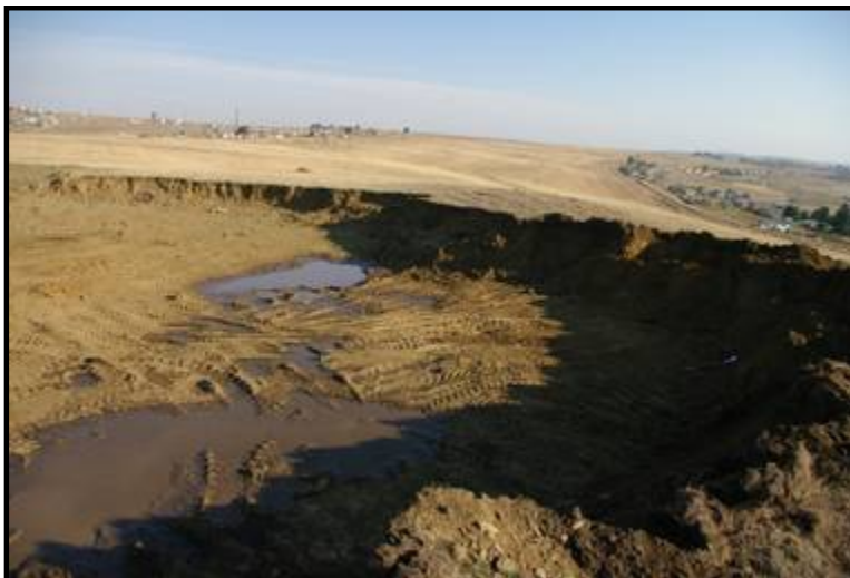
Figure 19: View of a portion of the borrow pit 290_BP01 study site
