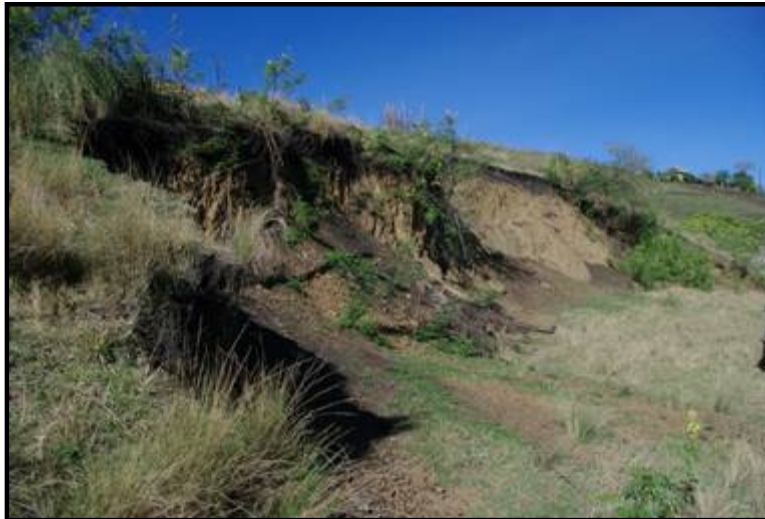
Figure 77: Current impact at borrow pit 151_BP01
